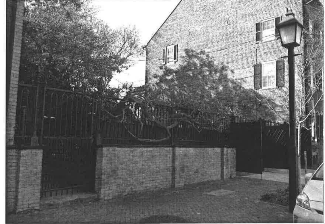
View from Prince Street: cast iron fence on 4' ht. brick wall (now painted). Fence was likely installed by the bank in the late 19th century.
