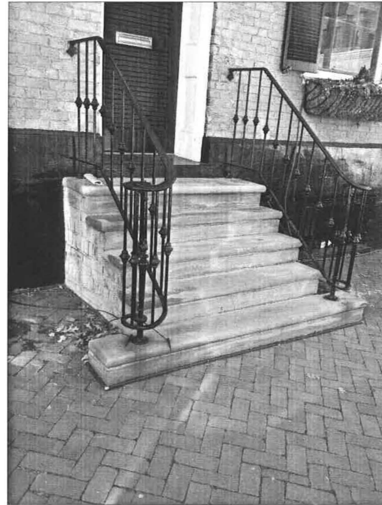
Modern steps and rail at front door.
