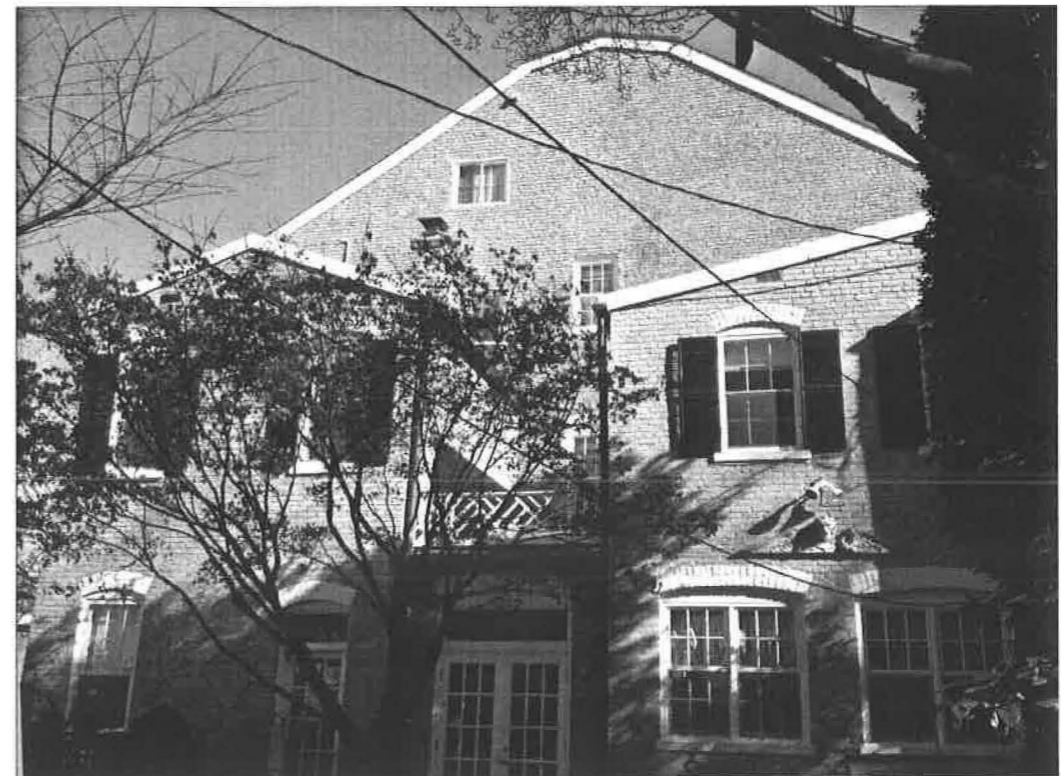
View from garden of west ells and first floor infill between; west wall of main block above/beyond. Note windows on ells and west side of main block are modern.
