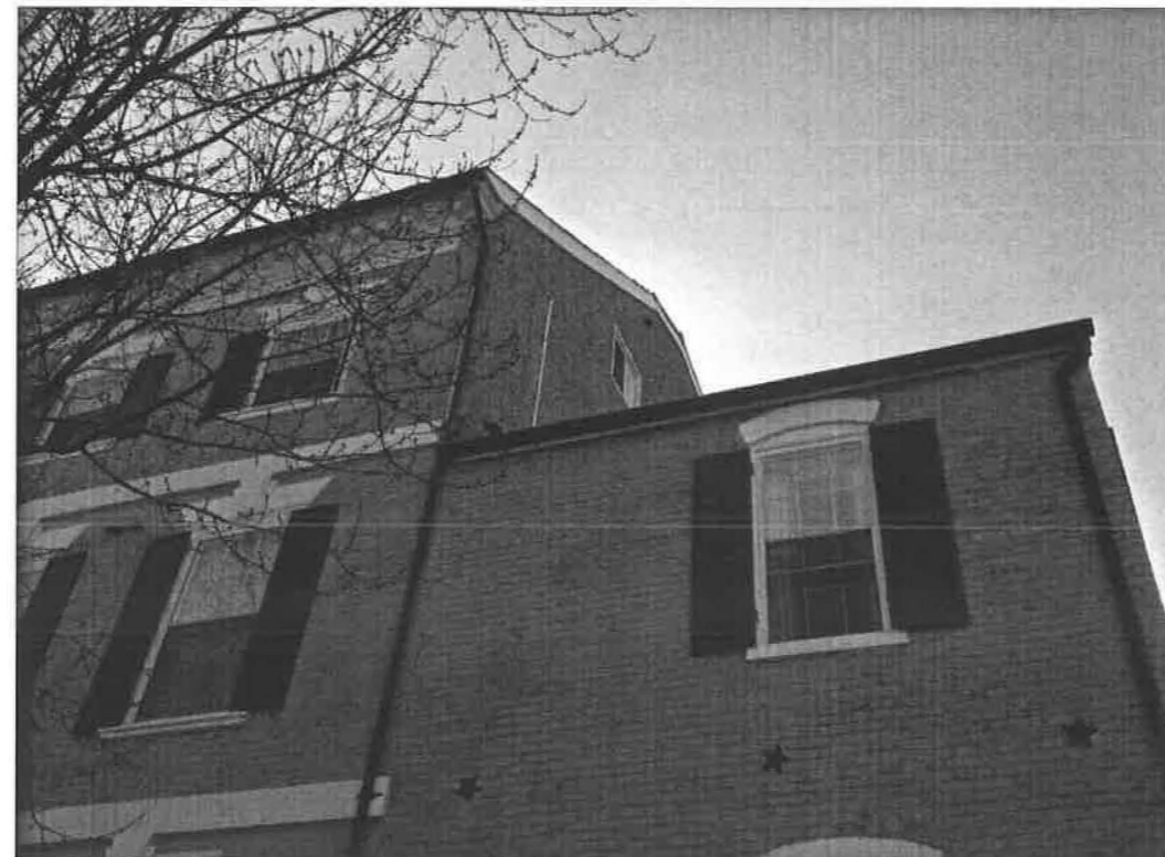
West ell at north side as viewed from Prince Street
