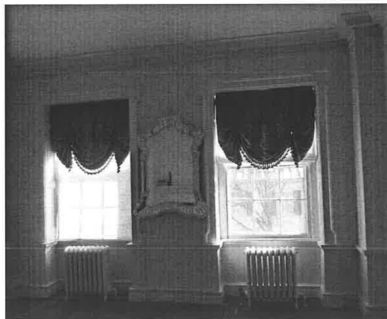
2015 - 2nd floor Hooe Parlor replacement
