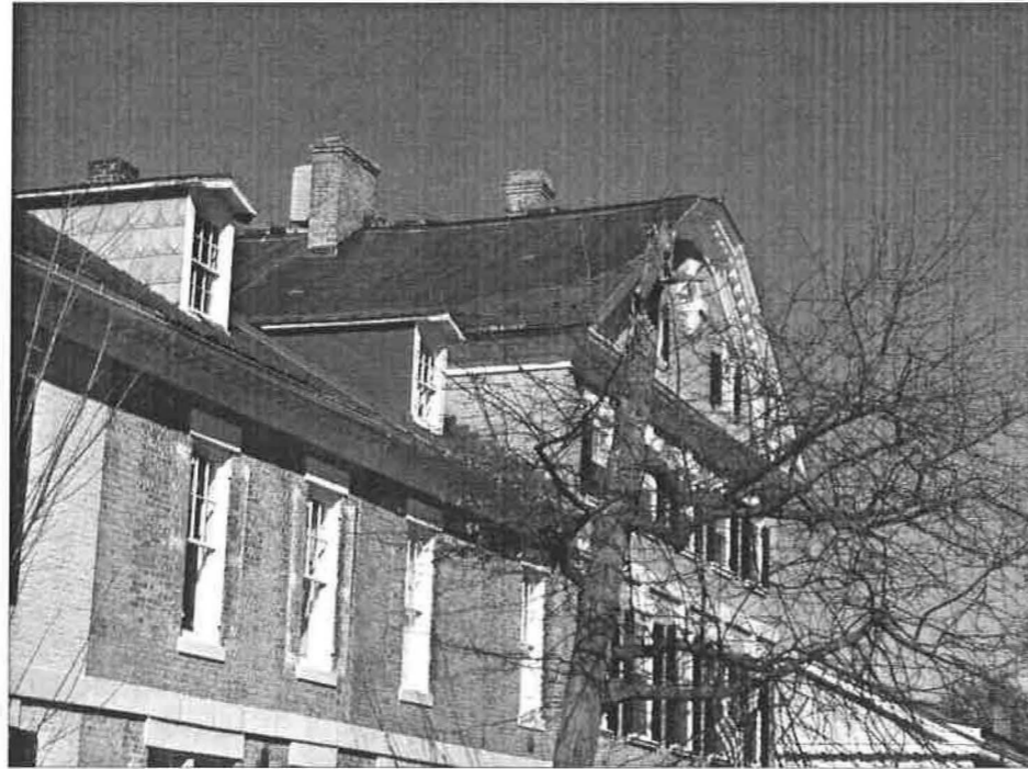
View of c. 1780 south wing - original to house. Much altered in 1910 after a fire and converted into rowhouses.
