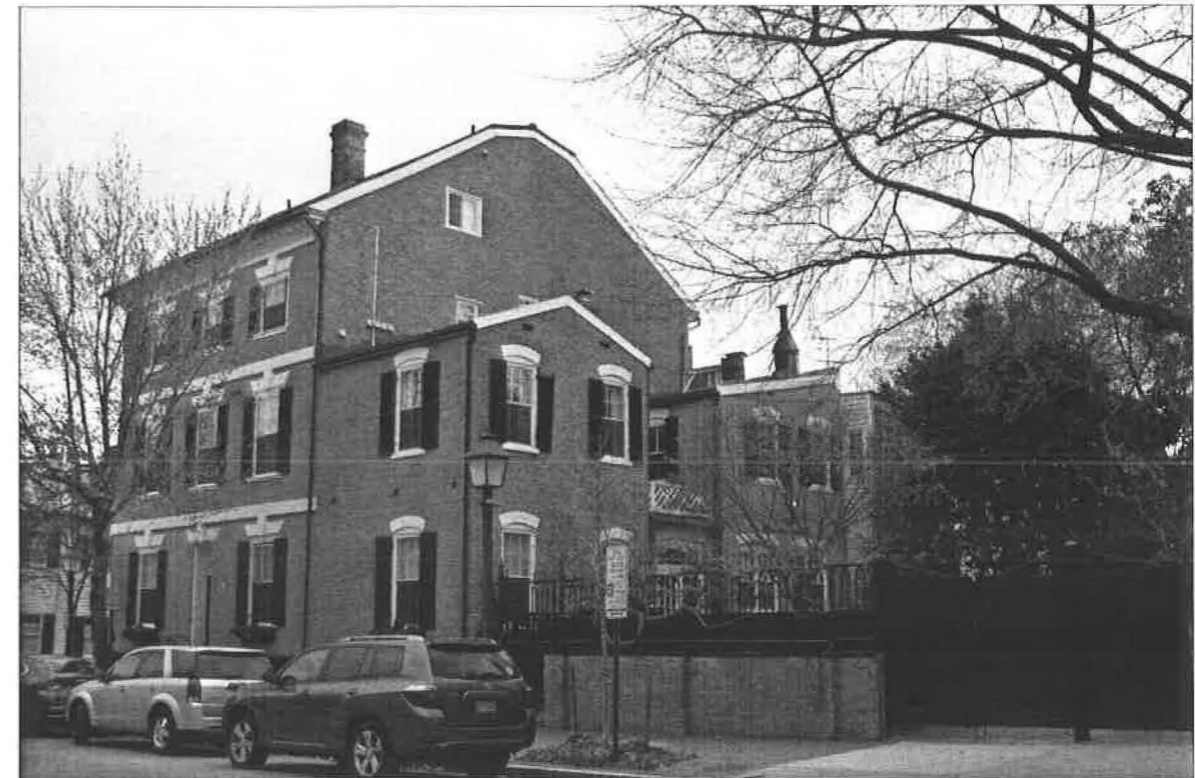
View from Prince Street looking southeast. Note ells built to west of the Hooe House constructed in 1910 for the duplex conversion. Windows at ells are modern 6/6 replacing original 2/2.
