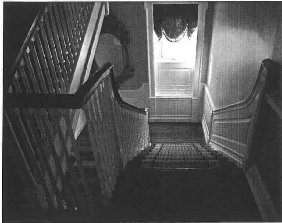
2015 - 2nd to 3rd floor stair landing. Woodwork to be replicated for restored 1st to 2nd floor stair.
