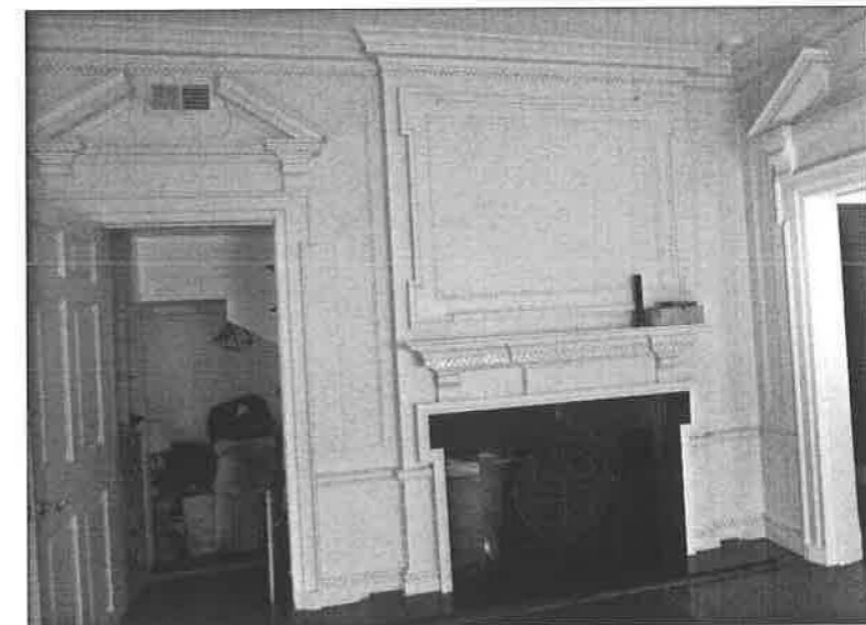
2015 - 2nd floor Hooe Parlor replacement
