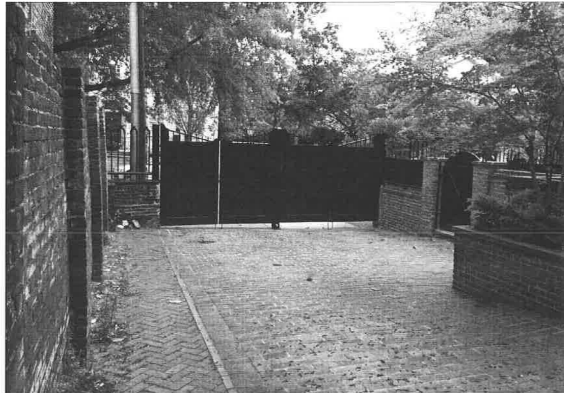
Parking Area with gate to Prince Street, looking north. Note: modern painted wood gates to drive will be removed.
