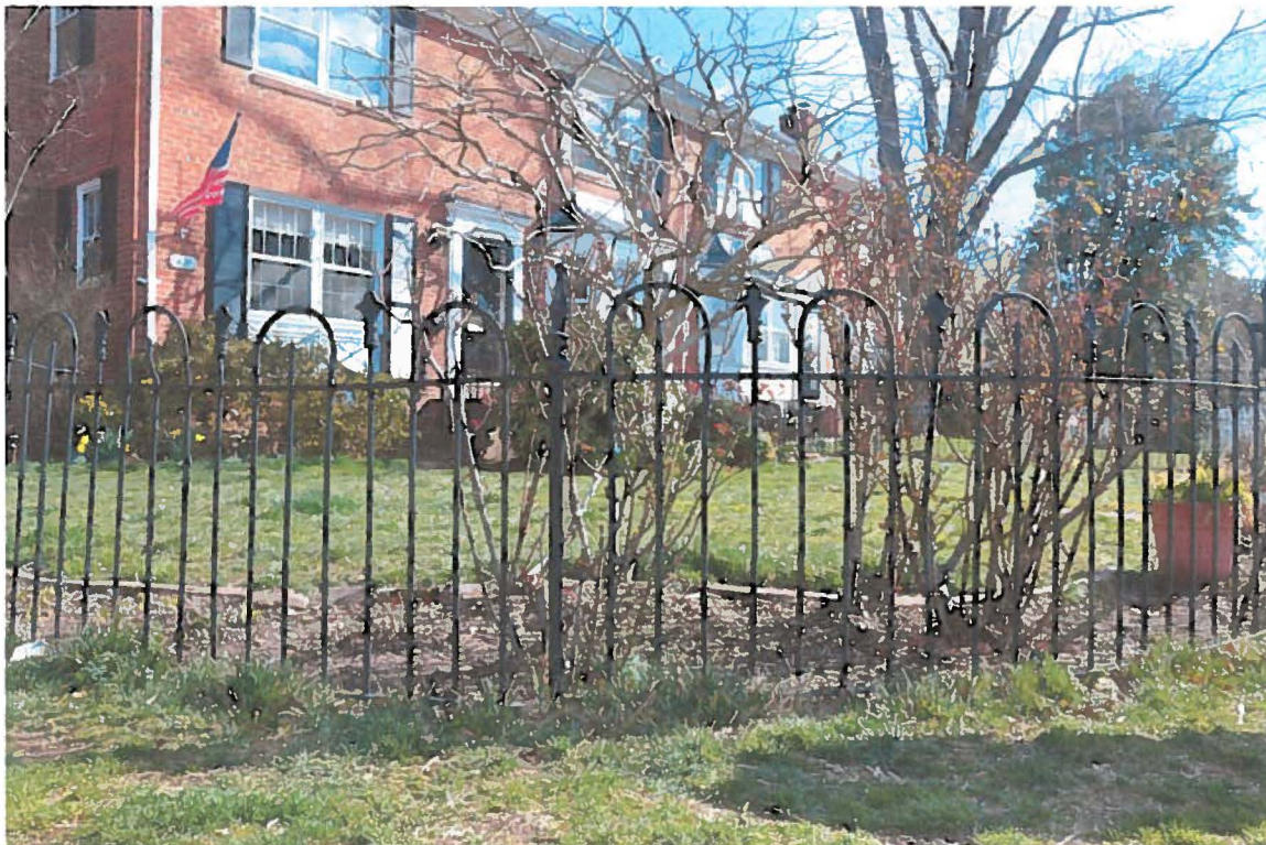
Adjacent Neighbor's Ironwork
