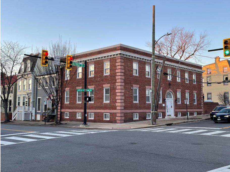
Figure 7 - South and East elevations view from the intersection
