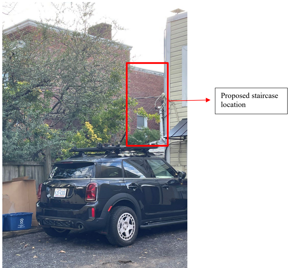
Figure 4 - rear/west elevation view from alley
