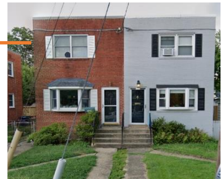
Two-story dwelling. (105 A&B E Del Ray Avenue)
