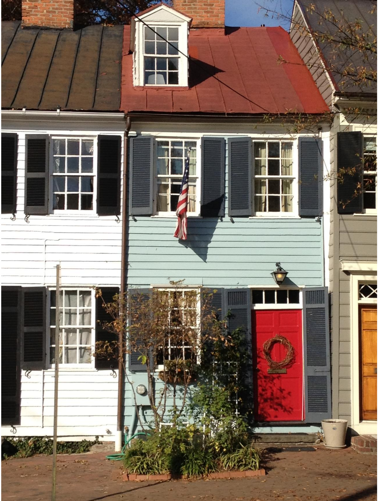
Front Façade – 323 Duke St.
