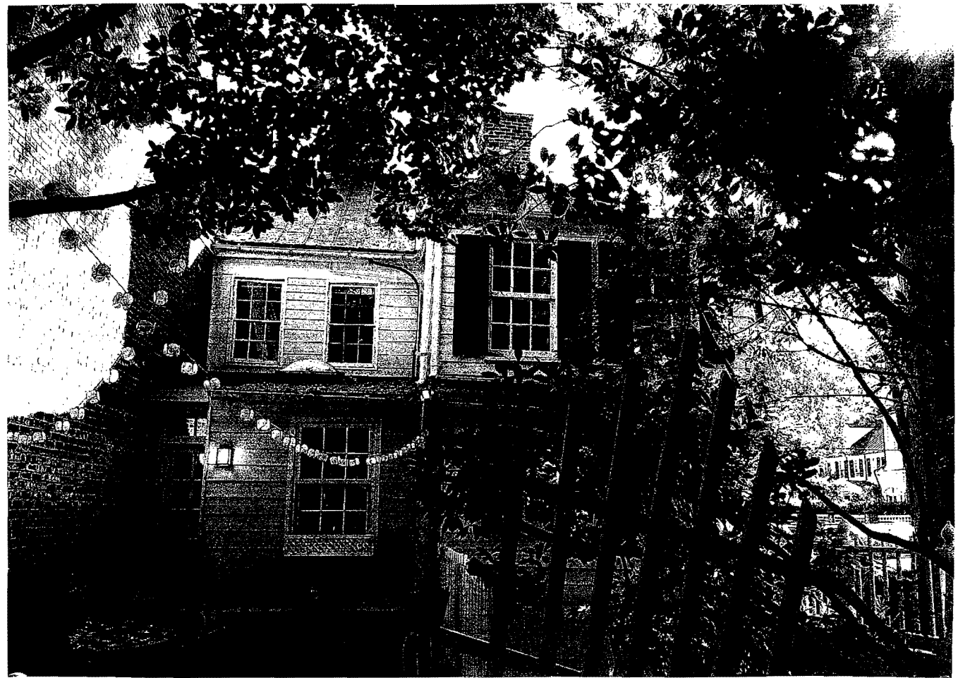
REAR OF 323 DUKE ST.
