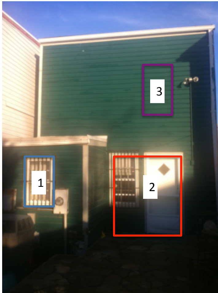
Figure 1: 708 N Patrick St. rear elevation (west facing)
