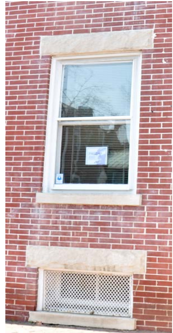
CLOSE-UP OF EXISTING DOUBLE HUNG WINDOW & BASEMENT WINDOW W/ GRILL
