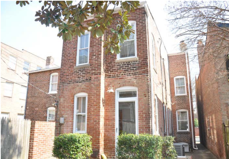
REAR ELEVATION SHOWING ORIGINAL 2 OVER 2 WINDOWS
