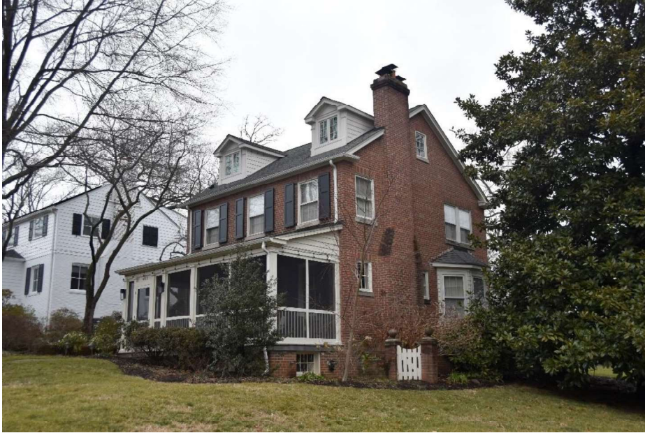
Existing South Corner of House (with 403 Jackson Place seen in the background)
