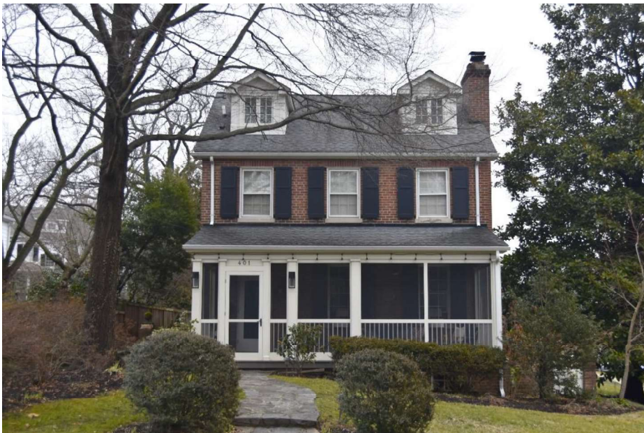
Existing Front of House (southwest side)
