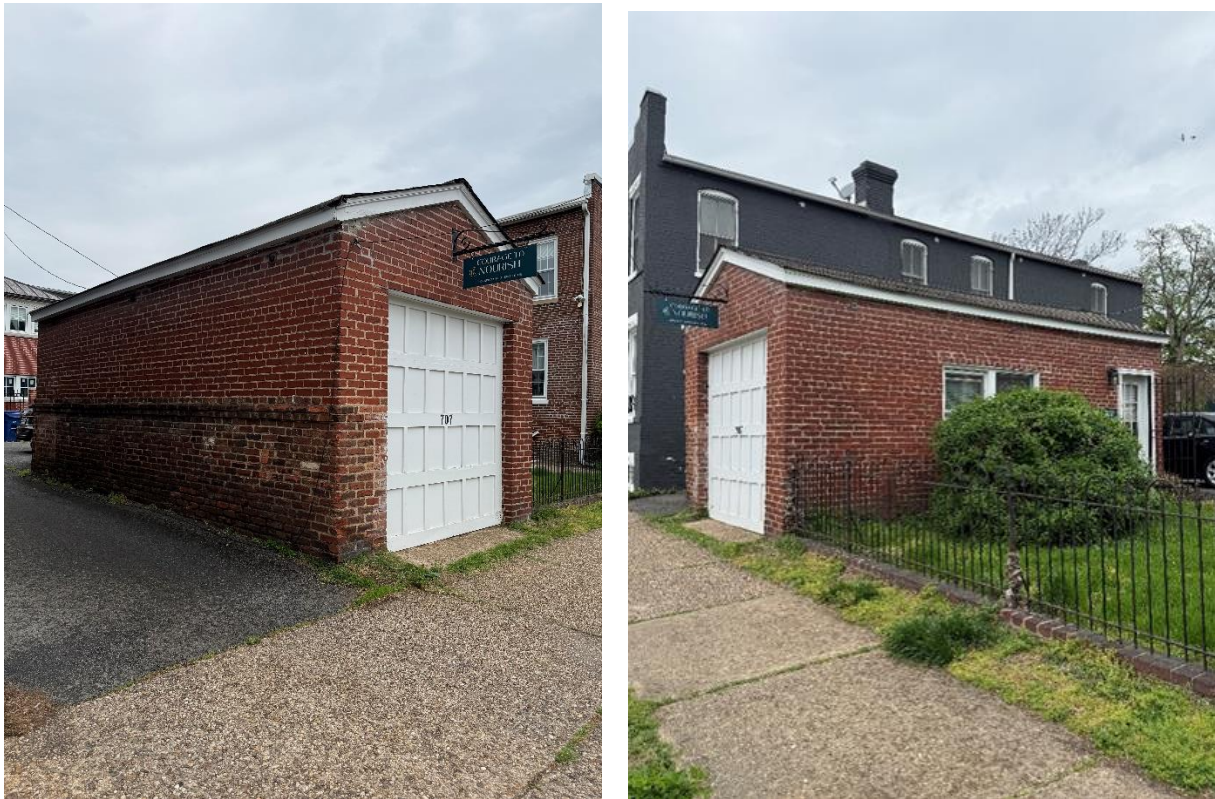
Figure 1 and 2 - Ancillary building to be demolished
