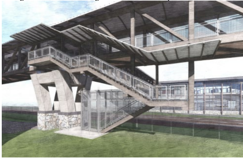
Figure 12: View of egress stair showing roof mass and railings
