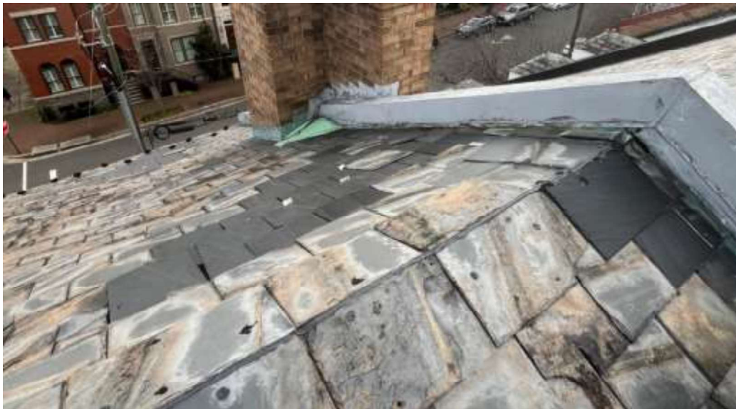
Figure 2. The condition of the existing roof.
