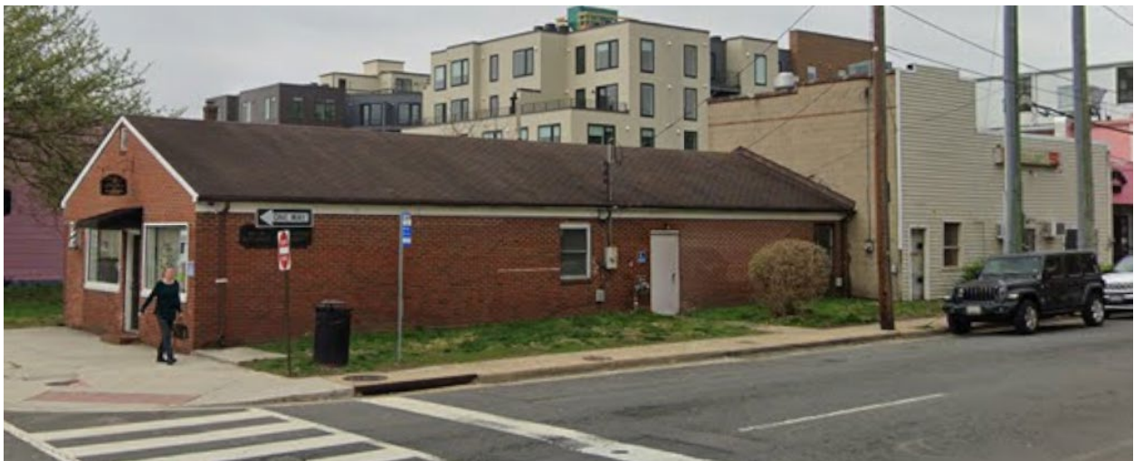
Figure 1: Buildings at 728 N Patrick and 1006-1008 Madison to be demolished
