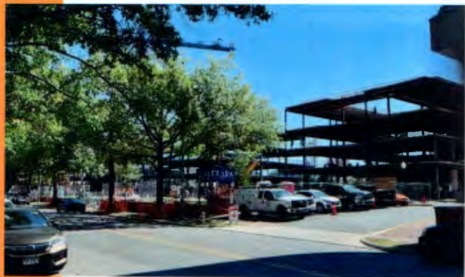
Site under construction, summer 2024
