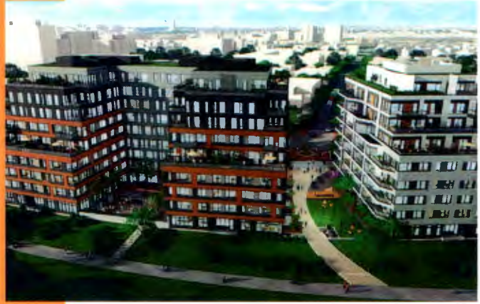
View of entire site from east elevation
