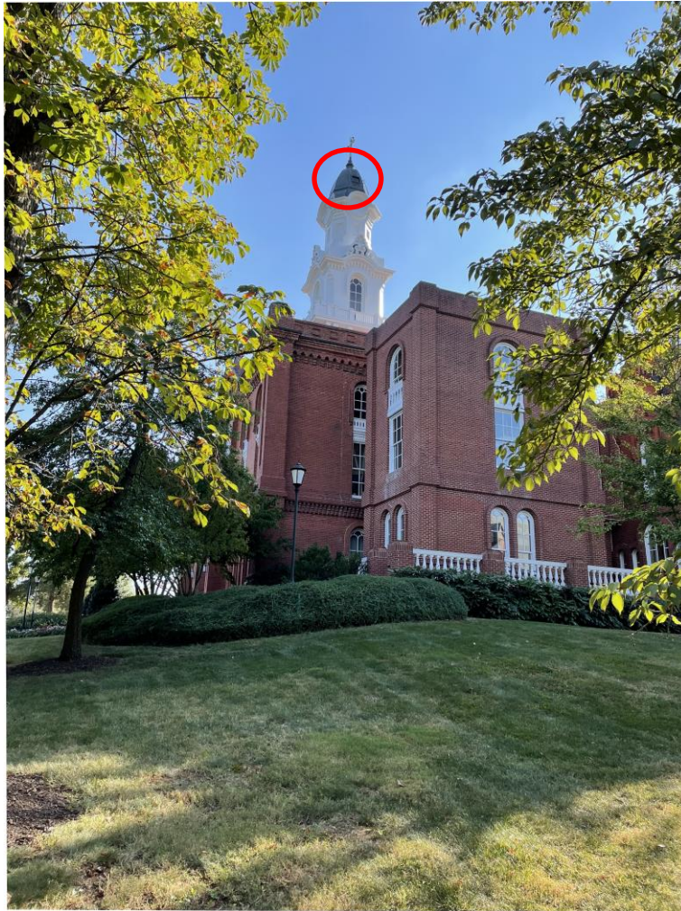
Figure 2 - Existing hatch visibility
