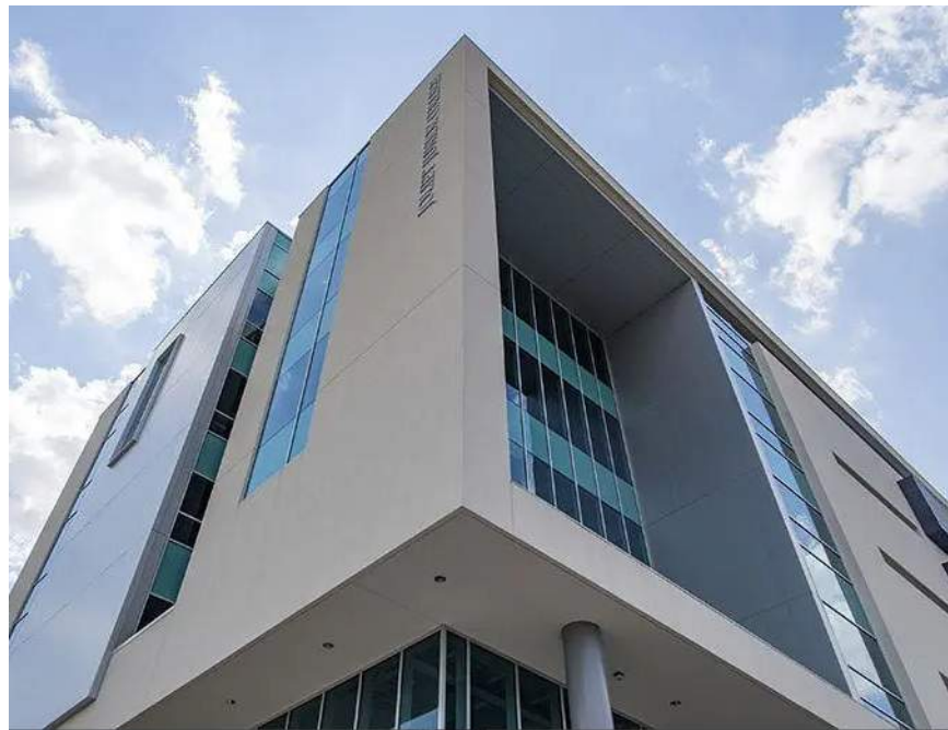
FIBER-CEMENT PANELS AT REAR/ALLEY: SHADES OF GRAY BY JAMES HARDIE ("HARDIEPANEL"), USING METAL TRIM PIECES AT CORNERS AND PANEL JOINTS, AND BREAK METAL AT OPENINGS.
