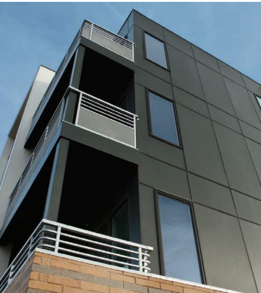
FIBER-CEMENT PANELS AT REAR/ALLEY: SHADES OF GRAY BY JAMES HARDIE ("HARDIEPANEL"), USING METAL TRIM PIECES AT CORNERS AND PANEL JOINTS, AND BREAK METAL AT OPENINGS.
