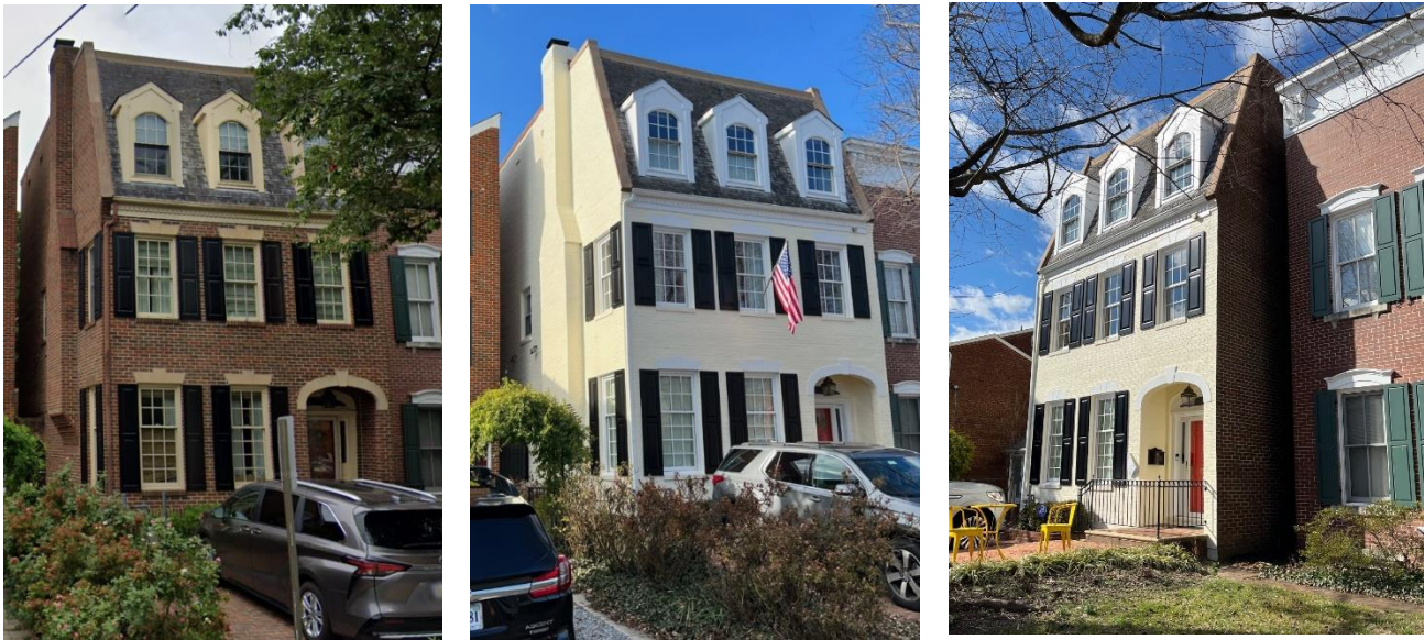
Figure 1. Photos of 613 S Royal Street before and after painting.
