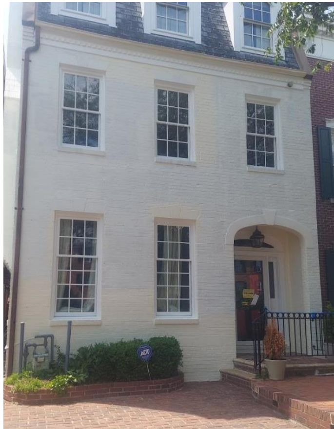
Figure 2. Photo of 613 South Royal Street after (partial) painting.
