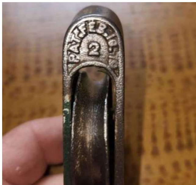
Figure 4: “Norris Pulley” similar to the one found in the subject windows.
