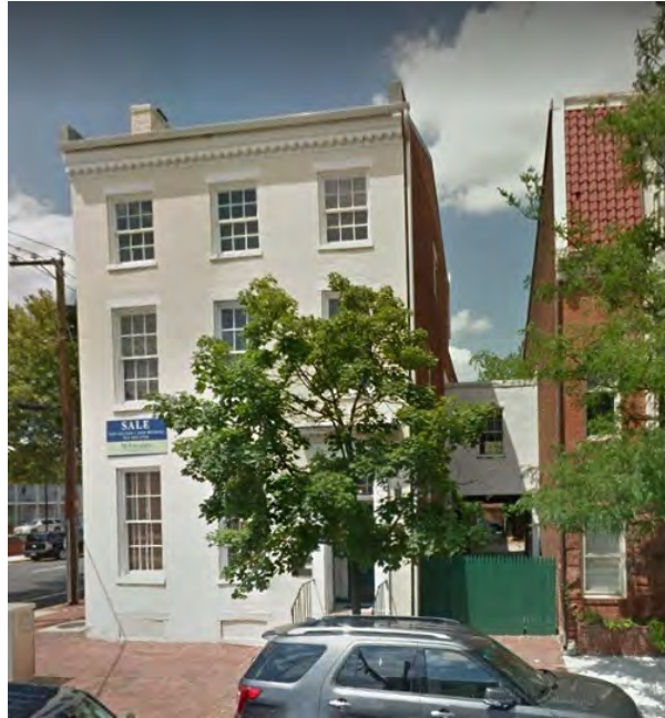
Figure 3: South elevation: notice gap under second story overpass on right. This gap will be enclosed.
