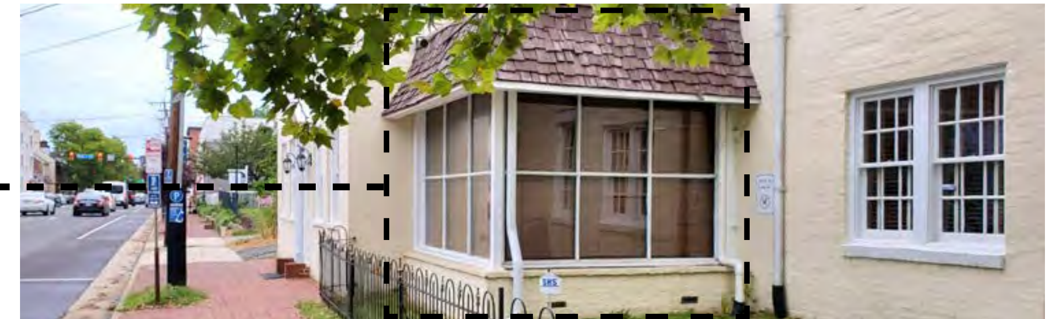
S. PATRICK FACADE [EXISTING DISPLAY STOREFRONT FACADE]
