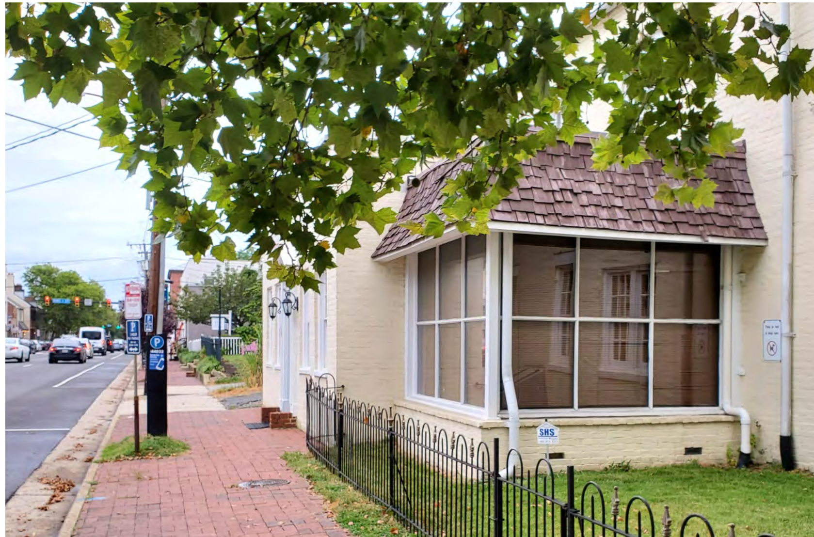
Patrick Street Storefront enclosure. The enclosure will be demolished to the masonry foundation.
