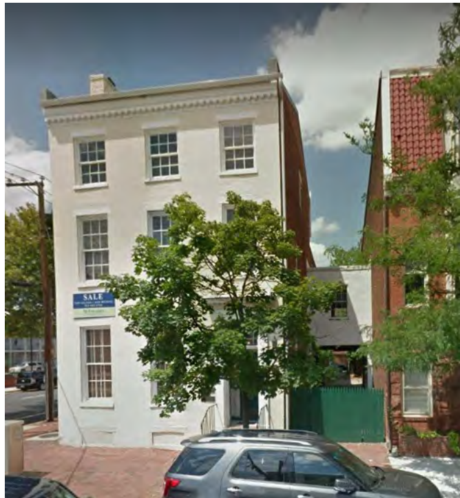
Figure 5: Existing south elevation
