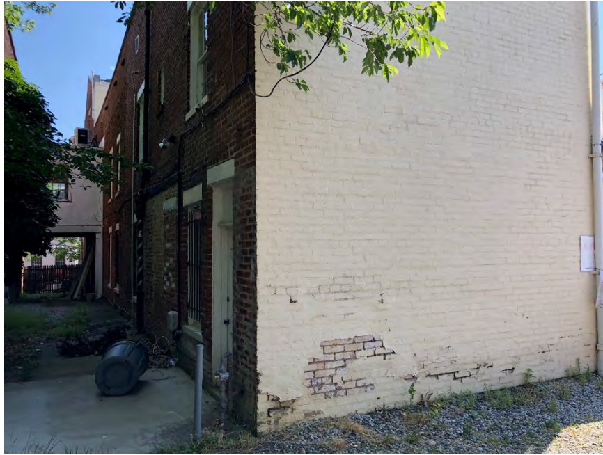
Figure 4: East elevation between 919 and 917 Prince Street showing existing conditions.
