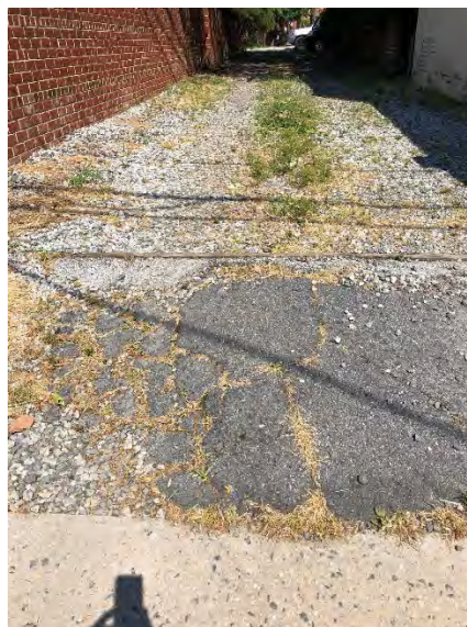
Figure 7: Alley to north of building existing conditions.
