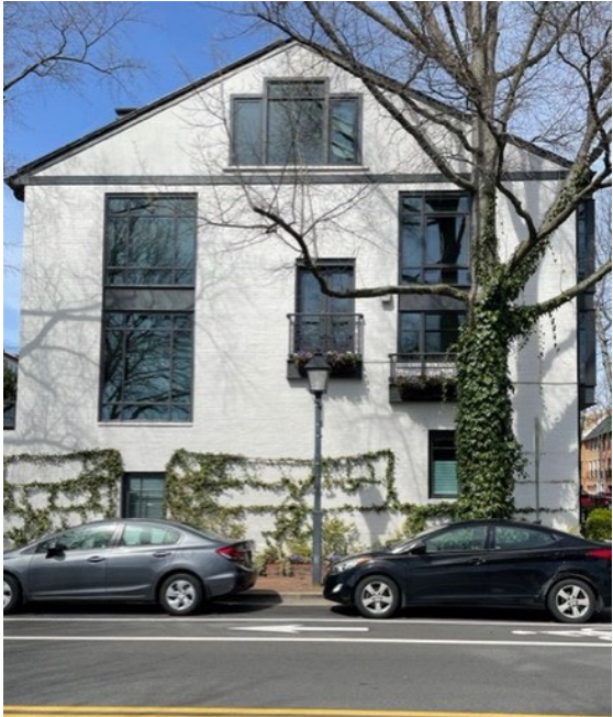
Photo 3 - 100 Quay Street east elevation
