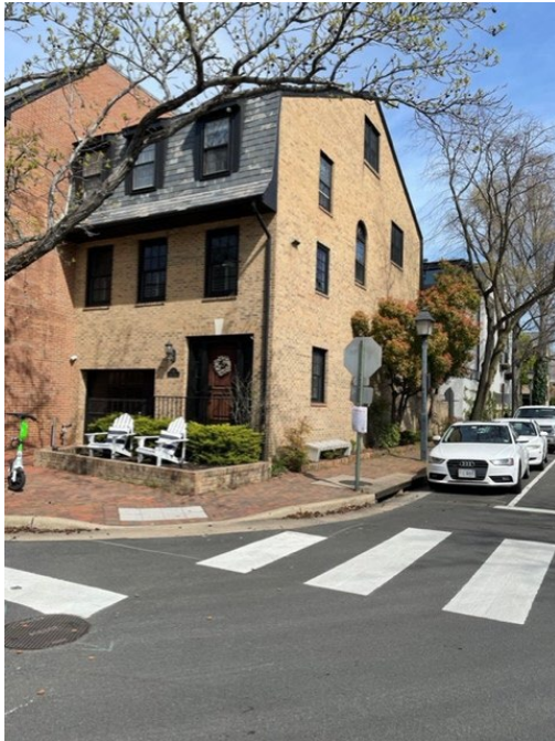
Photo 1 - South and east elevations
