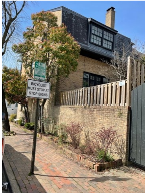
Photo 2 - North and east elevations
