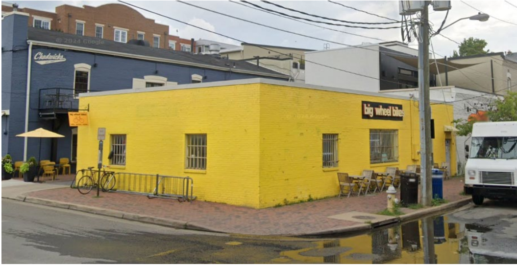
Figure 1: View of existing structure from the intersection of Strand Street and Prince Street
