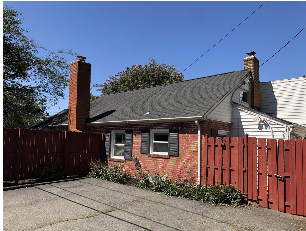
2. 1413 MT. VERNON AVE SIDE AND REAR FACADE
