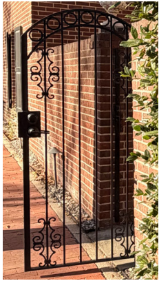
PHOTO OF EXISTING GATE TO BE REUSED
