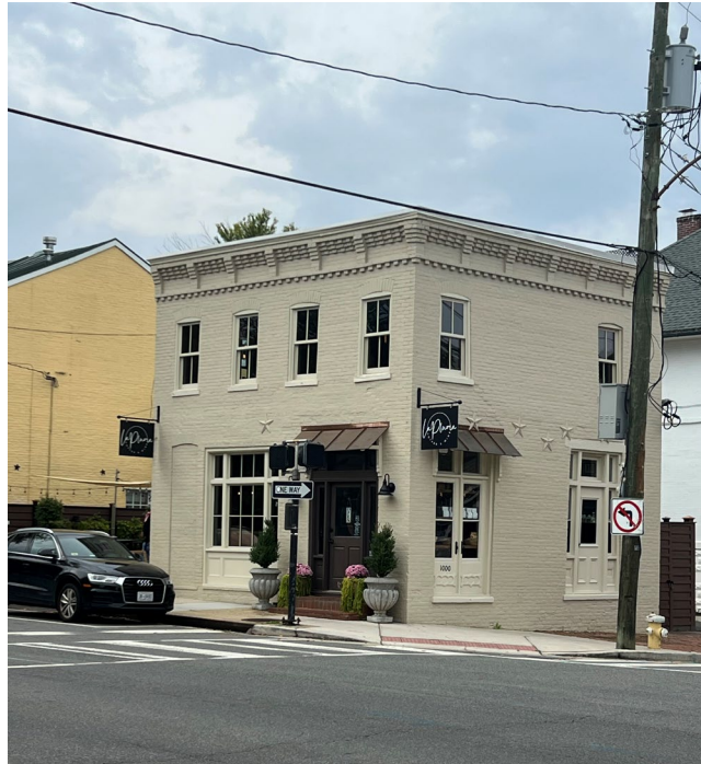
Figure 1: 1000 Cameron Street restaurant, La Pluma Coffee & Wine
