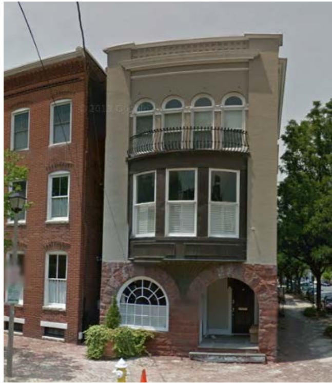
Bay window on a three-story house at 228 N. Columbus St.
