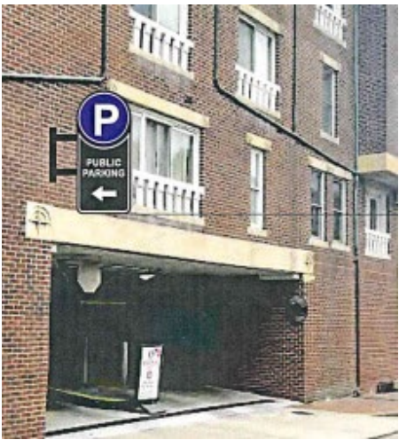
Figure 2: North Lee Street entrance
