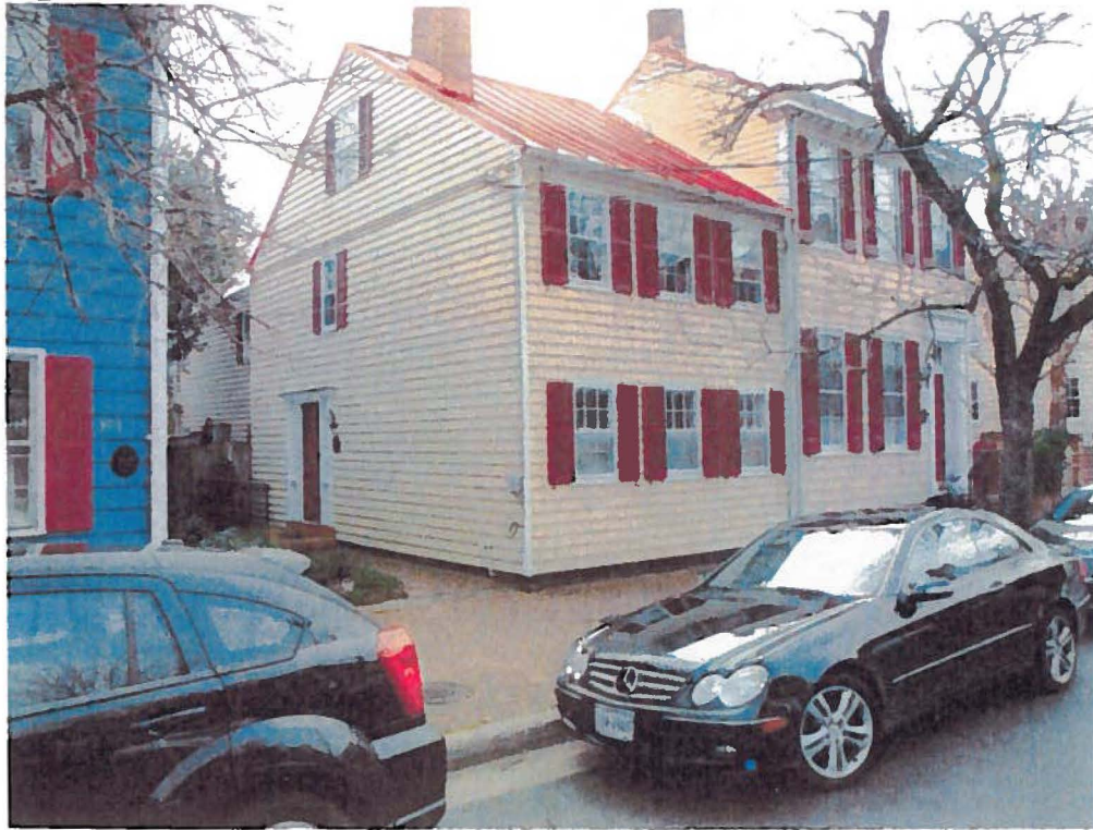
1 FRONT (WEST) FACADE FROM N. ST. ASAPH STREET Pic1
