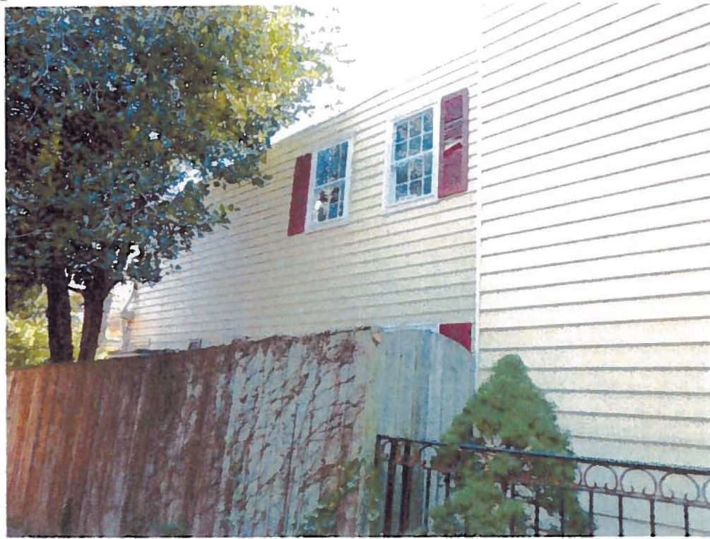
2 NORTH FACADE FROM SIDE ALLEY Pic1
