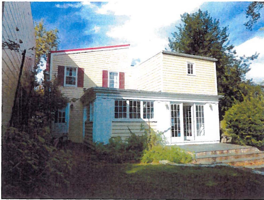
2 REAR (EAST) FACADE FROM BACK YARD Pic2
