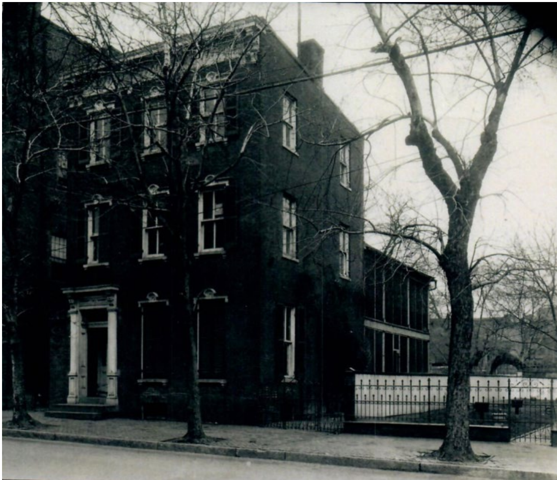
Figure 2: Vintage photograph of the structure at 411 Prince Street, showing early 2 over 2 windows
