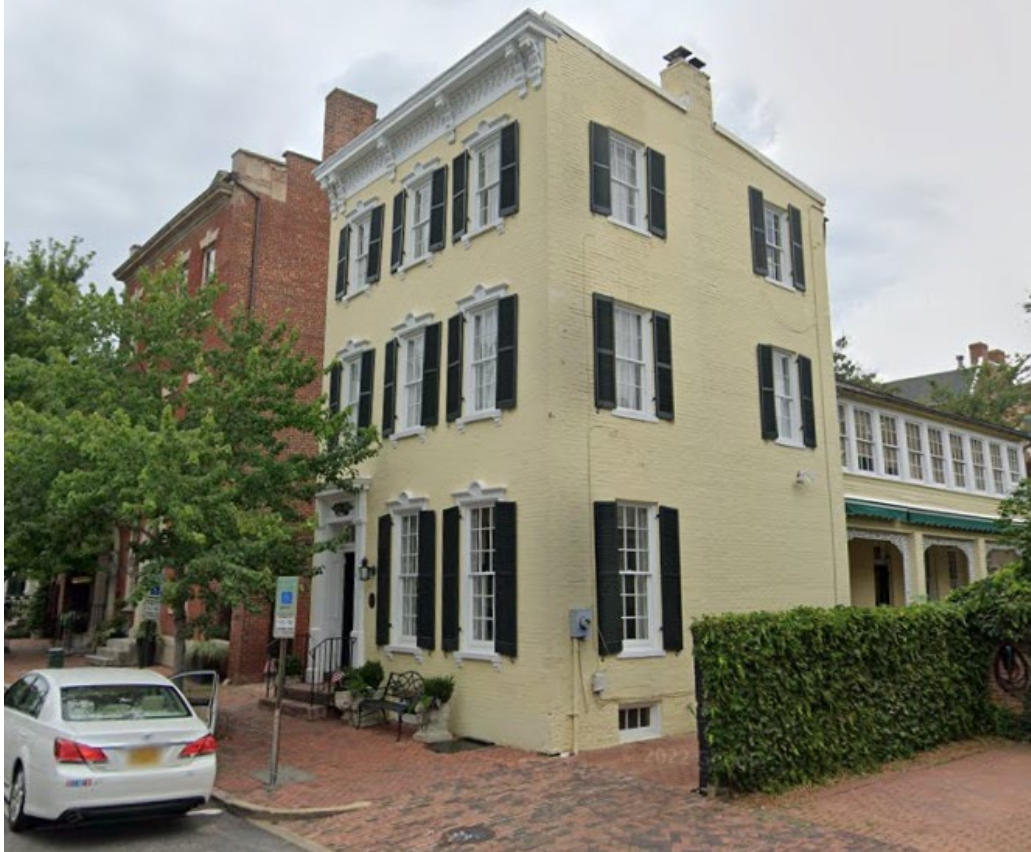
Figure 1: Windows on front portion of structure at 411 Prince Street to be replaced
