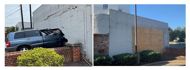
Figures 3 & 4. The masonry wall on the north elevation was damaged by a collision.
