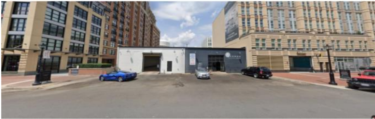
Figure 4: As part of a separate City Council lease agreement review, a new sidewalk section in front of Yates Auto Care will provide continuous and safe pedestrian passage along the 1000 block of North Fayette Street.
