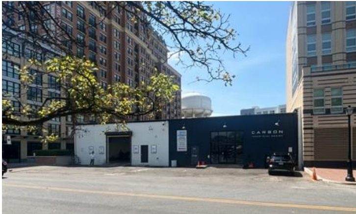
Figure 1: Front of Yates Auto Care on left at 1050 North Fayette Street.
