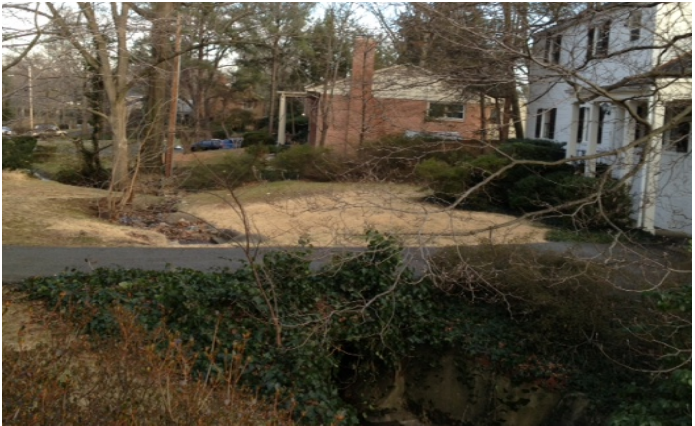
CULVERT AT 1412 KEY DRIVE...FRONT YARD
