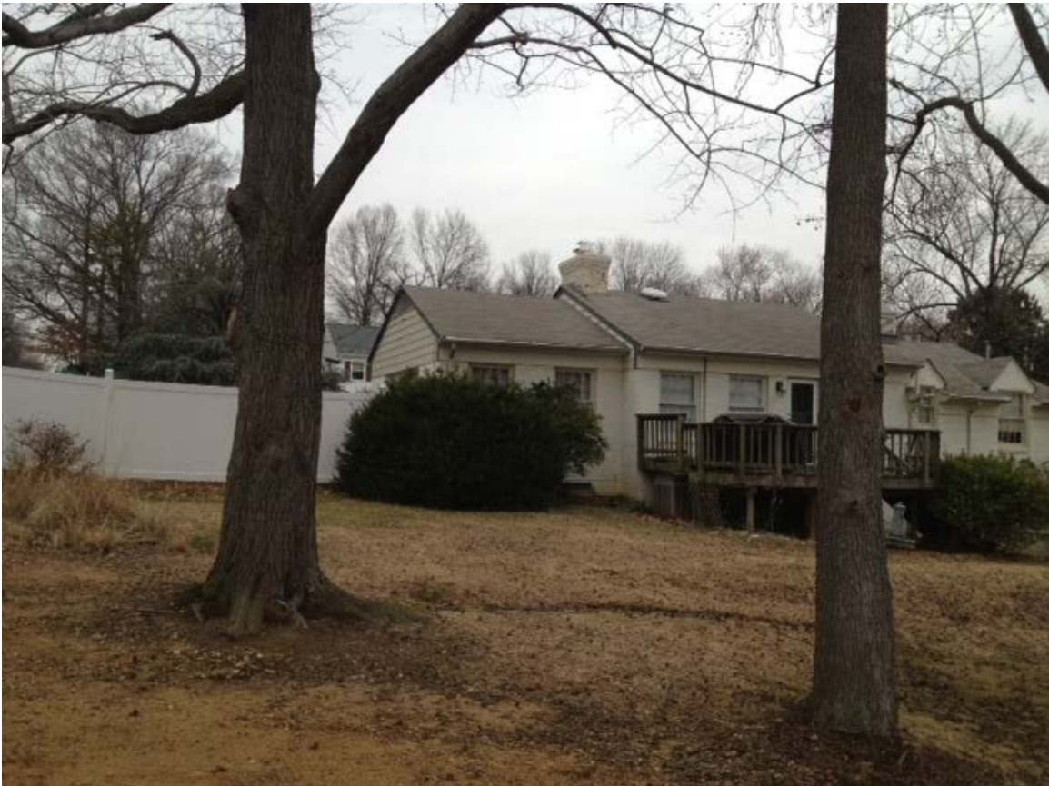
BACK OF OUR HOME FROM SW CORNER (THE BUSH IS WHERE THE PROPOSED HVAC/GENERATOR WOULD BE PLACED)
