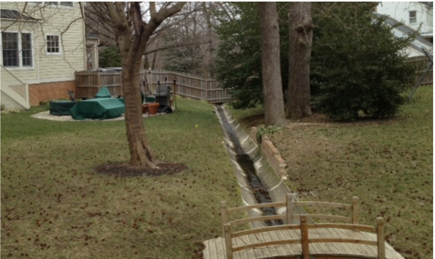
CULVERT AT 1416 KEY DRIVE...BACK YARD
