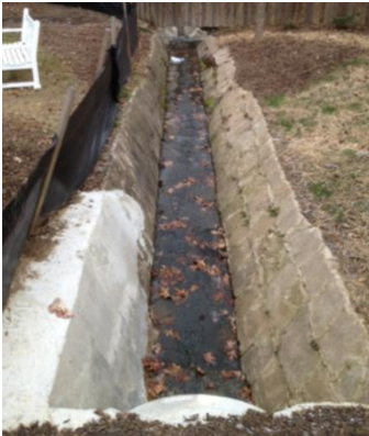
Culvert located across the southeast corner of the rear yard
