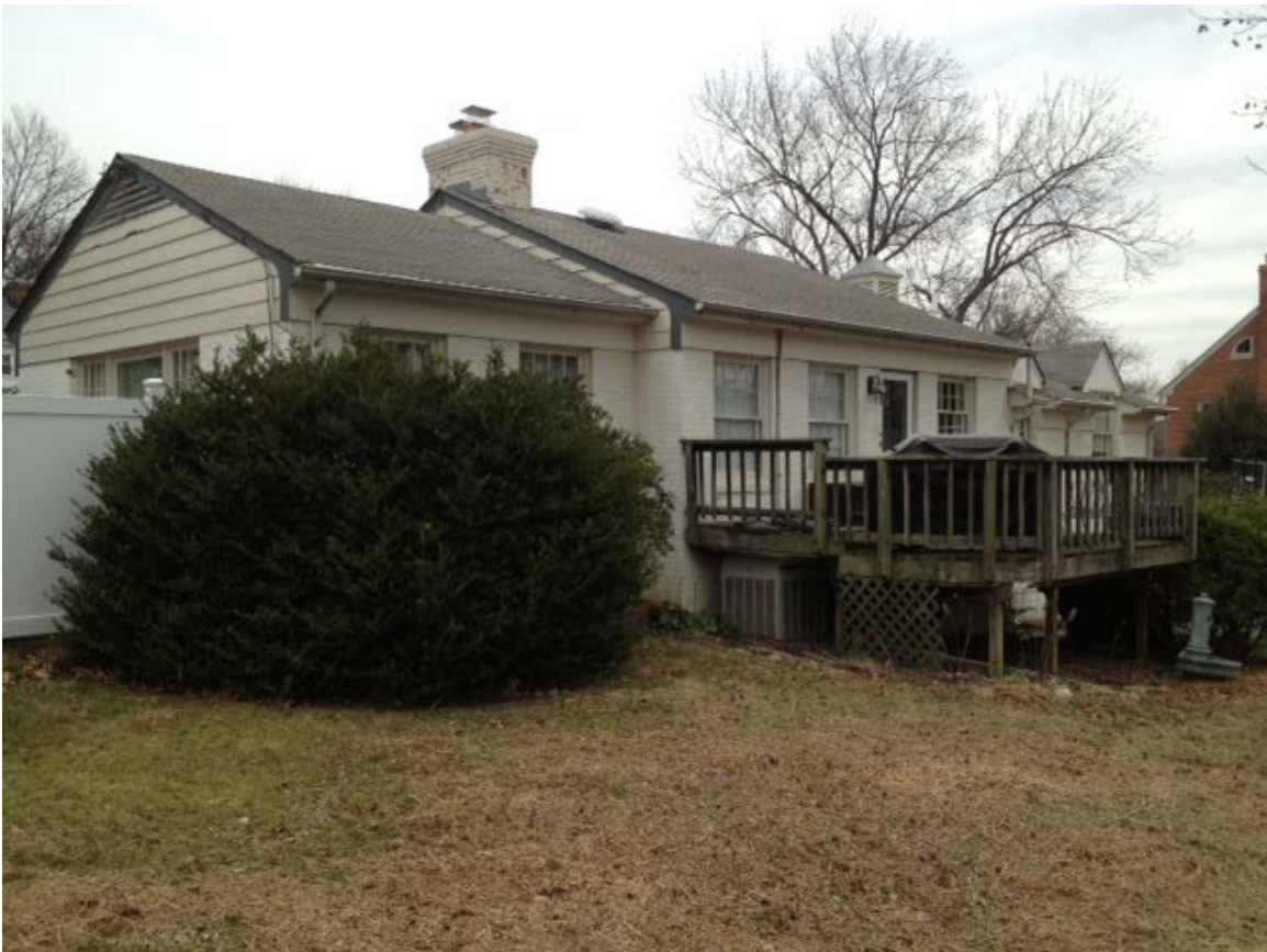
PROPOSED LOCATION OF OUR HVAC/GENERATOR
