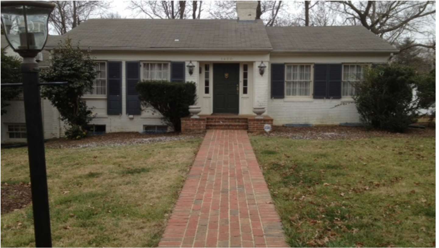
1420 KEY DRIVE (TAKEN FROM CURB FACE)
