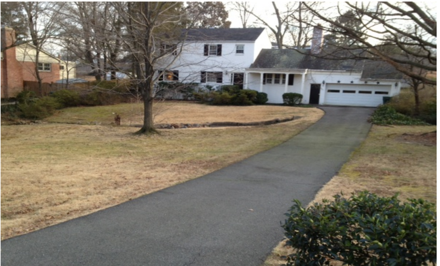
1412 KEY DRIVE (TAKEN FROM CURB FACE)
