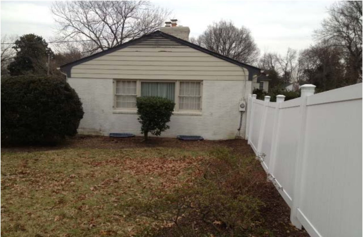
VIEW OF THE WEST SIDE OF THE HOME (BOXWOOD ON THE LEFT TO BE RELOCATED)
