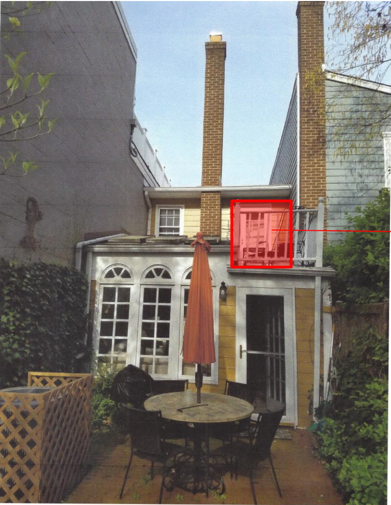
Figure 1 - Property rear/east elevation
