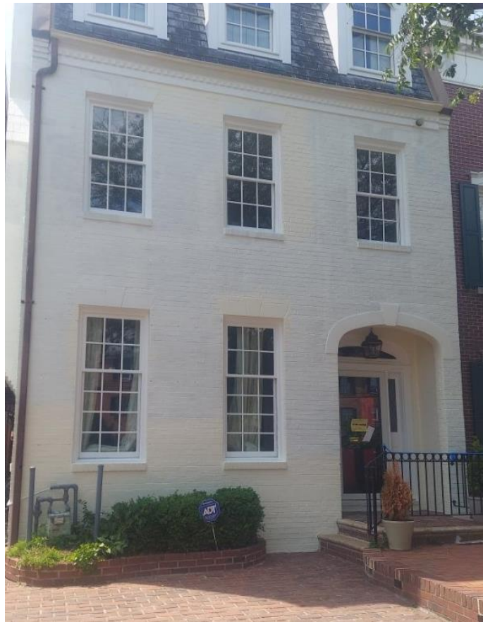
Figure 2. Photo of 613 South Royal Street after painting.
