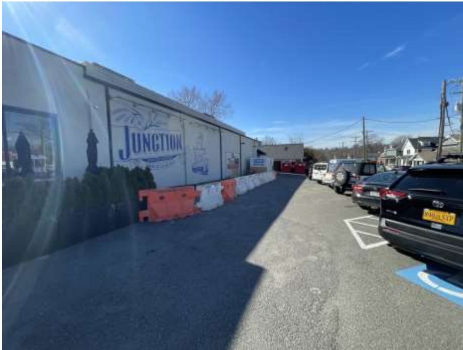
Figure 6: Future patio designated with barriers (left) and existing parking area (right)
