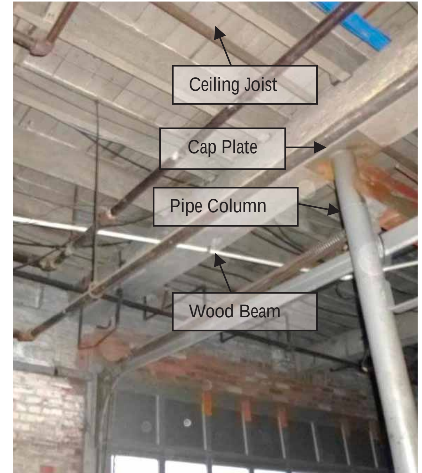
Interior Floor Framing
