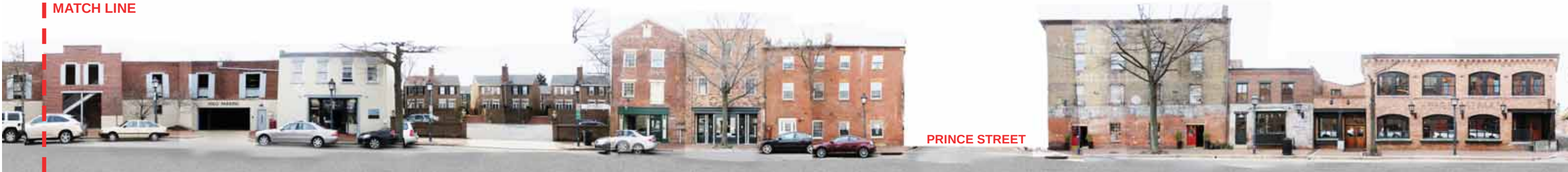
S. UNION STREET - LOOKING WEST (CONTINUED)
