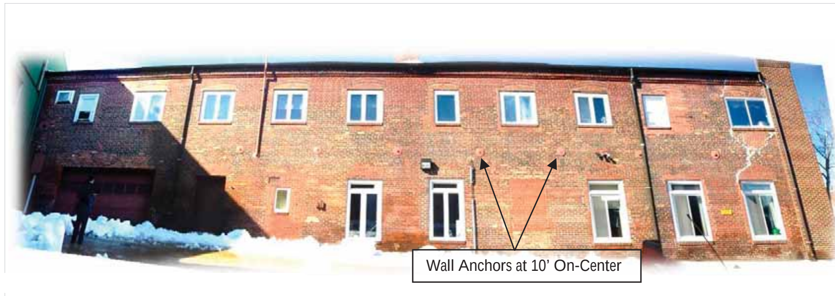
Masonry Bearing Wall Condition
