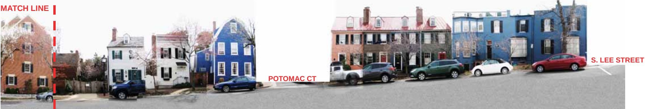
WOLFE STREET - LOOKING SOUTH (CONTINUED)
