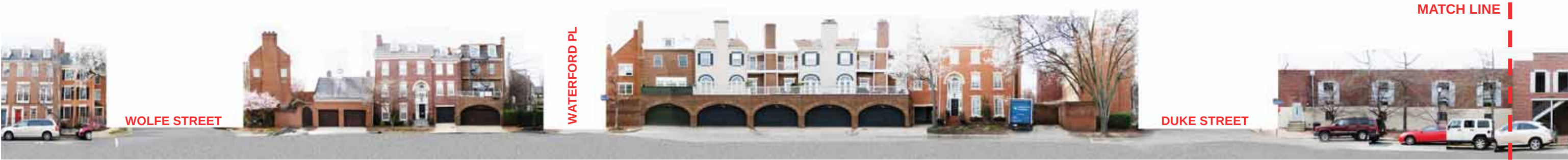
S. UNION STREET - LOOKING WEST
