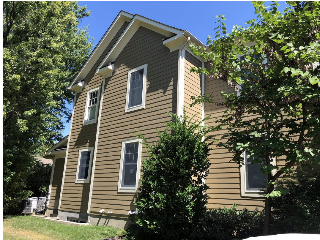
4. 408 E. ALEXANDRIA AVE. WEST SIDE YARD
