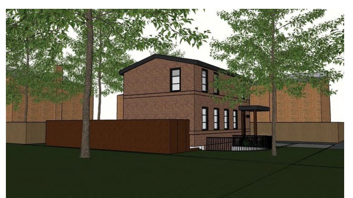
East Facade (side)
