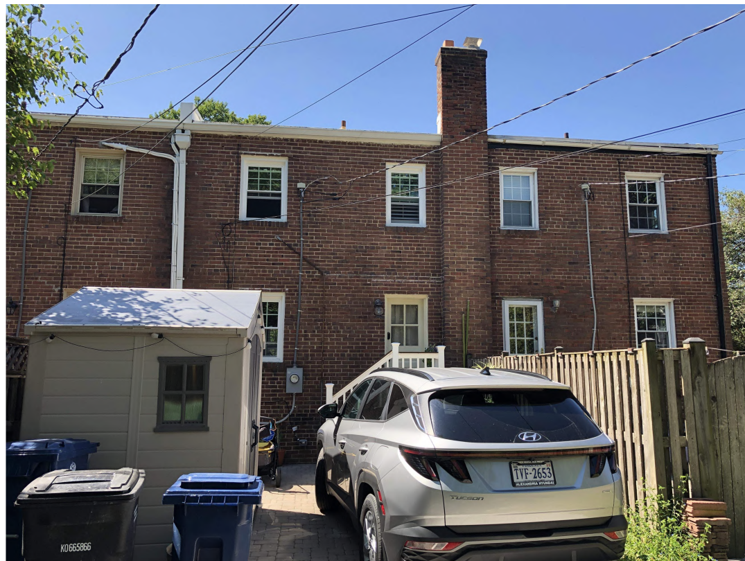
3. REAR FACADES AND YARDS OF 1407 - 1411
