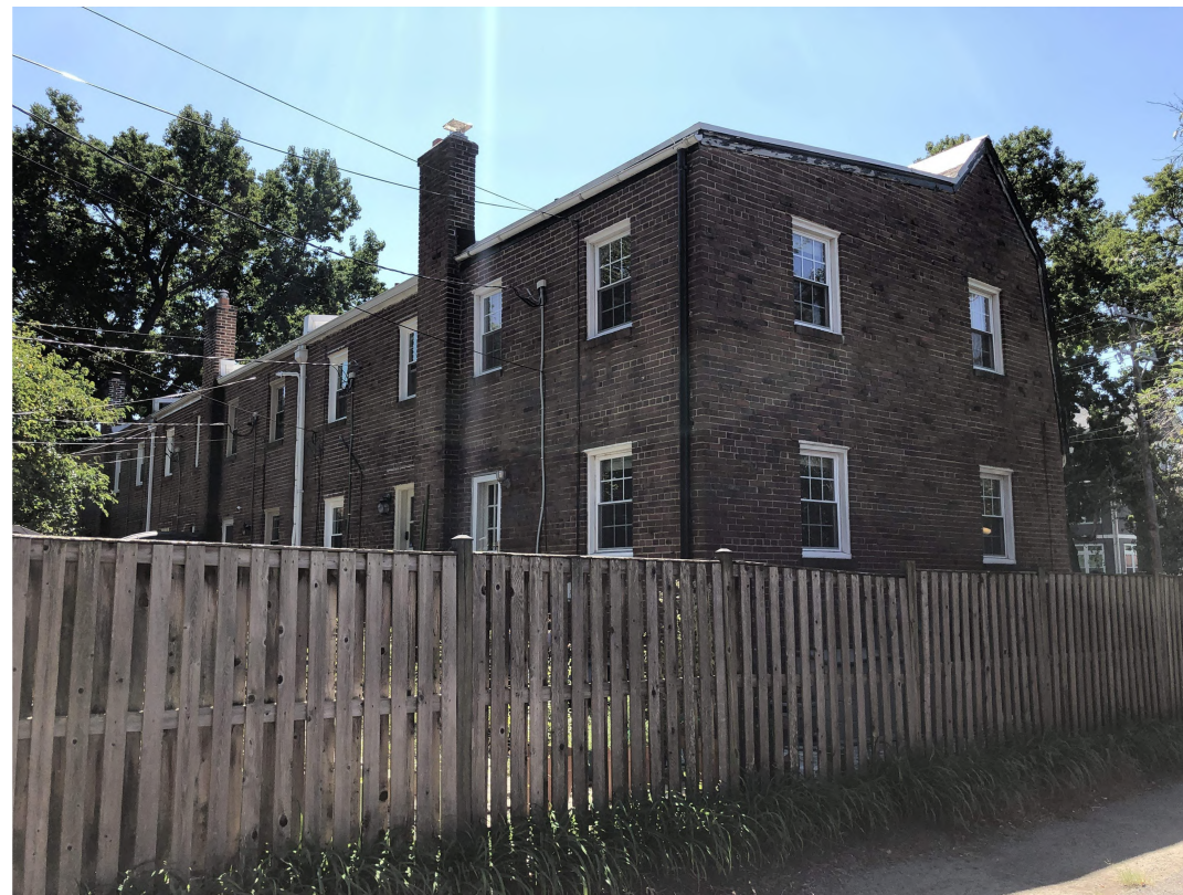
4. 1403 TO 1411 MT. VERNON AVE. REAR FACADES
