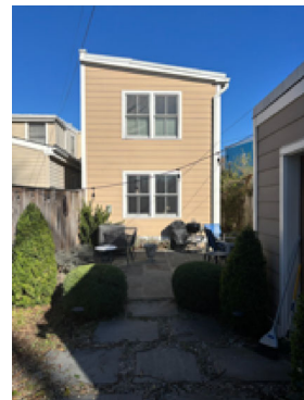
rear, inside fence
