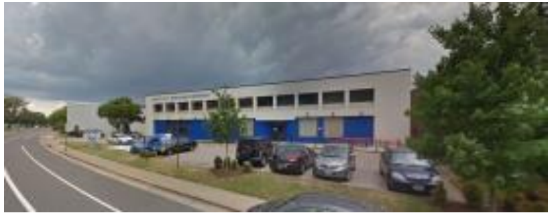
Figure 1: View of the site from Wheeler Avenue
