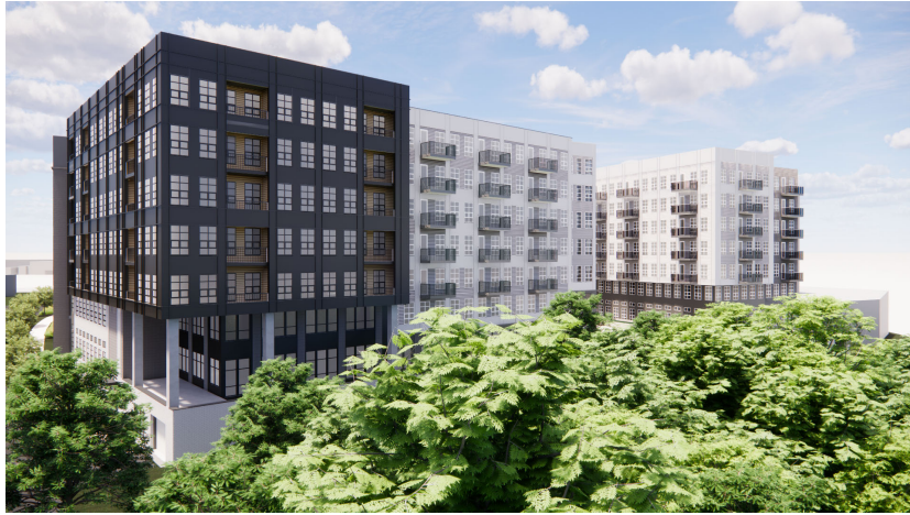
B4 | VIEW - NE CORNER
