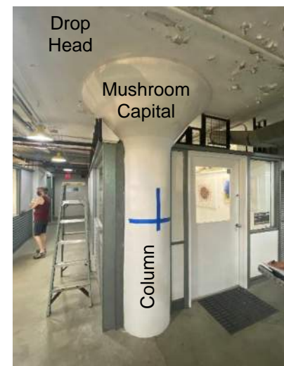
Fig 11 – Left: Schematic sections through Ground and 2 nd Floor Columns Right: Image showing typical column design with cylindrical shaft, mushroom capital and drop head
