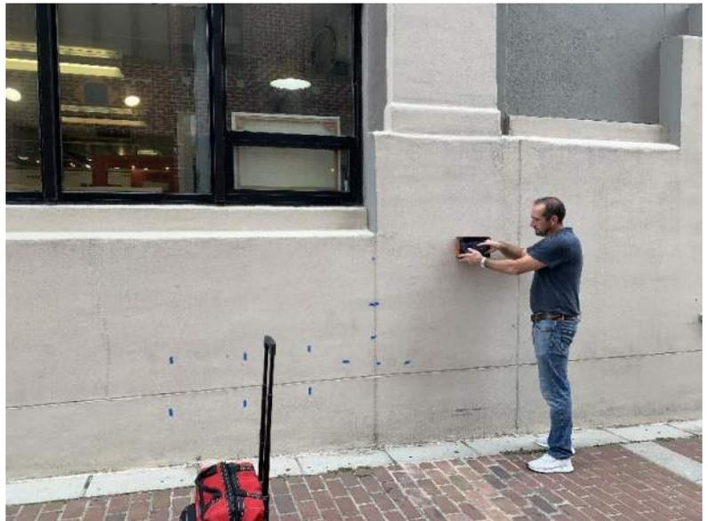
**Fig 6:** GPR Data collection through Exterior Wall
