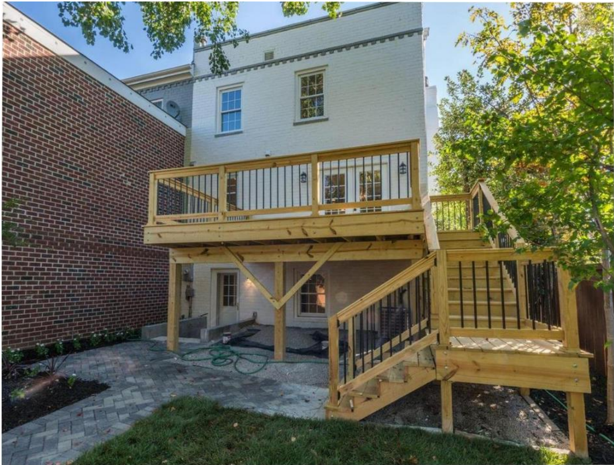
Figure 1 - Existing rear deck to be enclosed.
