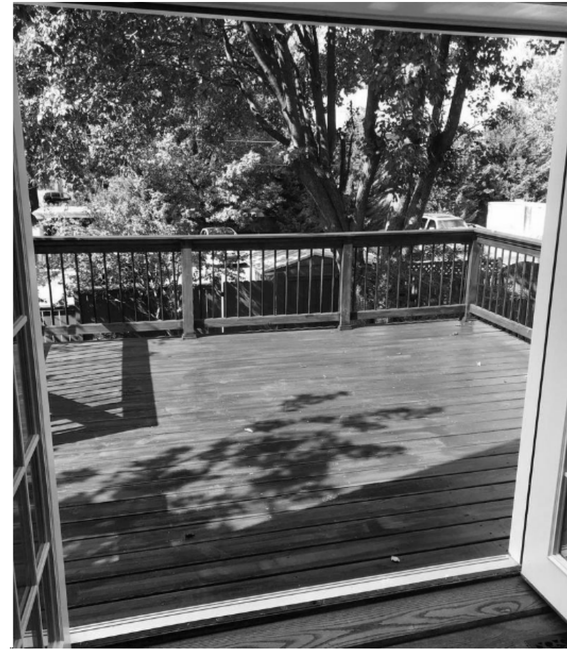
Existing Rear - From Interior
