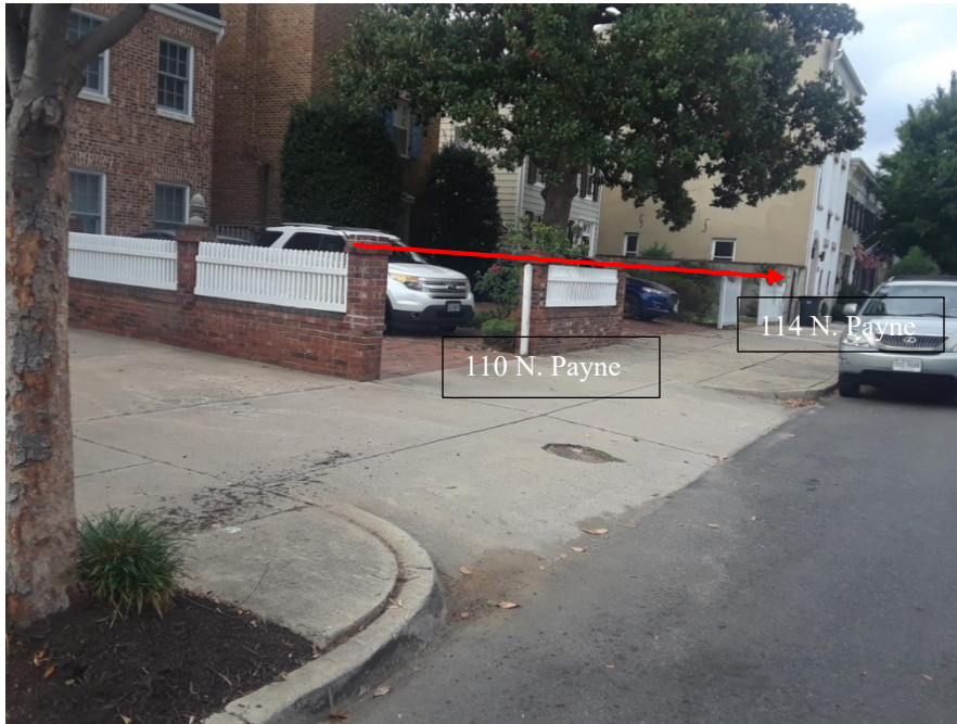
Figure 6: similar fence heights on the 100 block of North Payne
