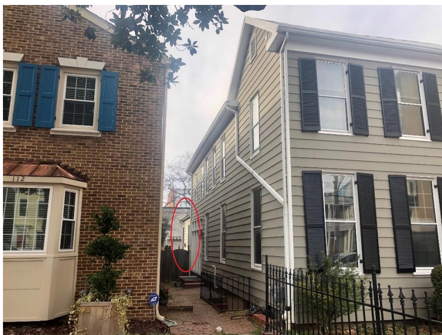
Figure 3: Southeast corner of house with existing one-story addition circled
