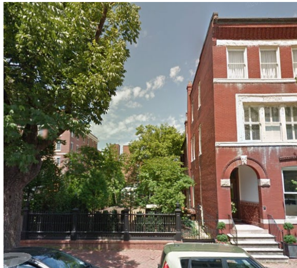
Figure 3: 805 Prince cast iron fence with masonry base
