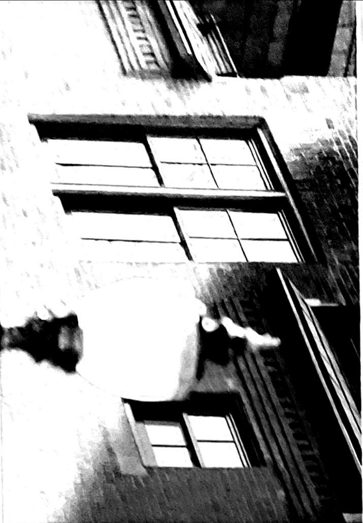
EXTENDED SASH LIPS SHOWN IN QUINCY, ILLINOIS PROJECT
