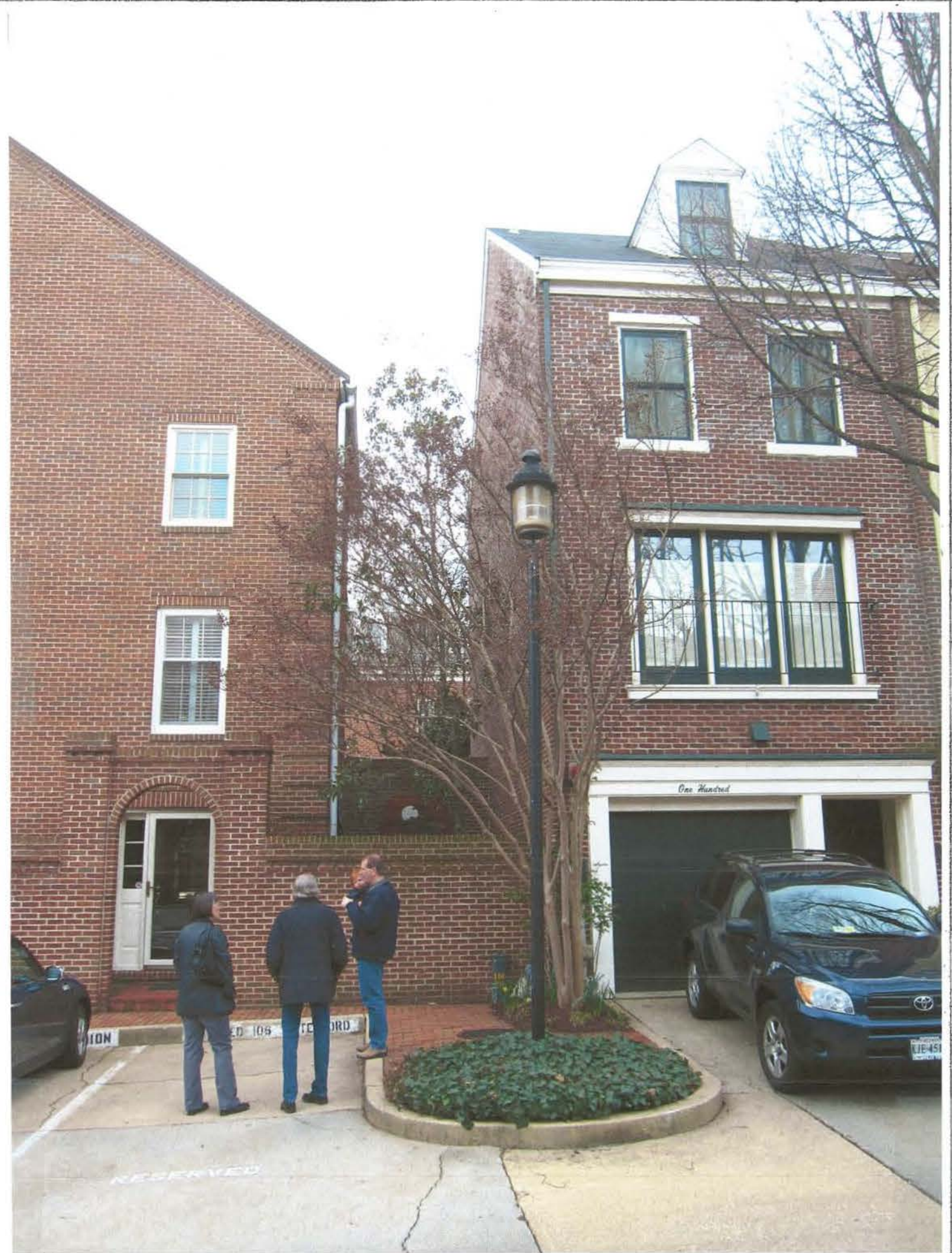
Existing NW Corner & Neighbor to West
