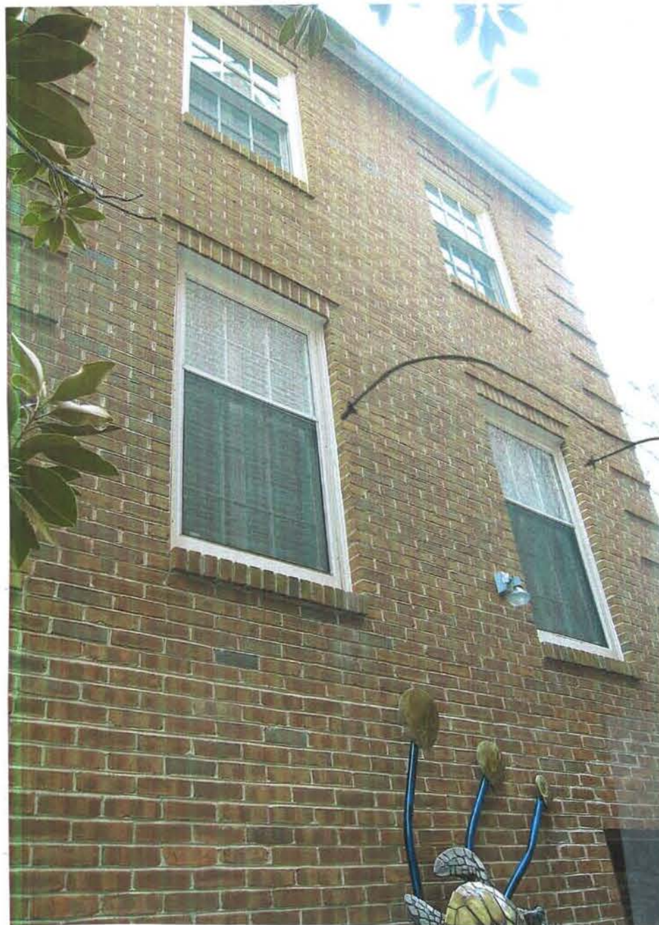
Existing Kitchen Windows @ West Face
