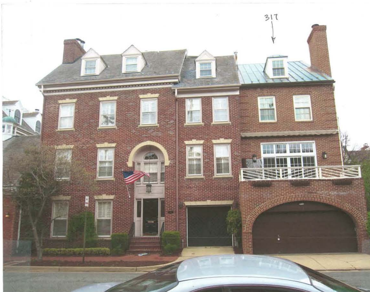
East Face of 317 & 319 S Union Street
