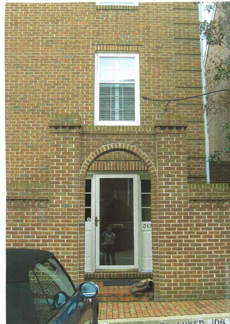
Existing Brick Piers & Kitchen Window @ North Face
