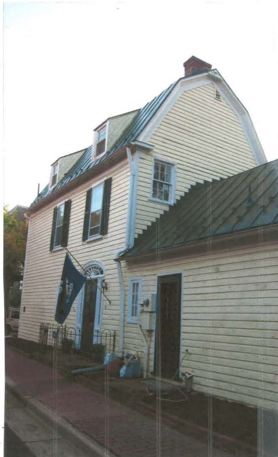
Gambrel roof at Wolfe & Potomac Court (historic)
