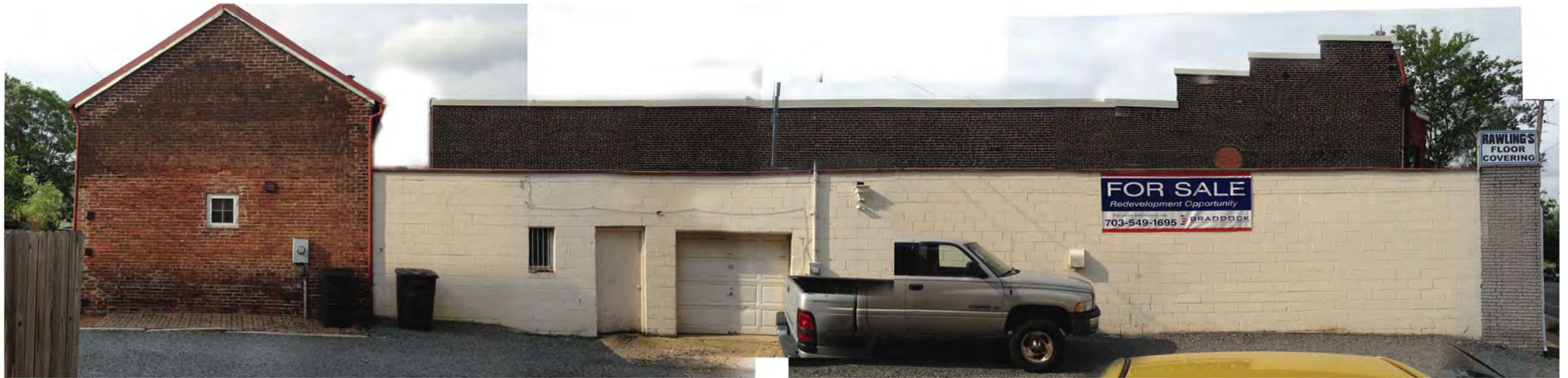
EXISTING NORTH ELEVATION VIEW FROM ALLEY
