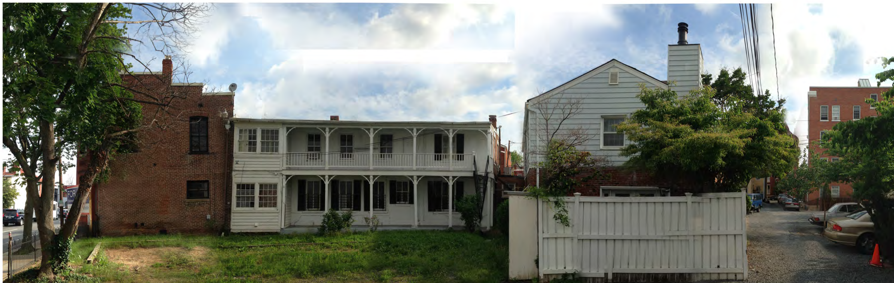
EXISTING SOUTH ELEVATION VIEW FROM VACANT LOT
