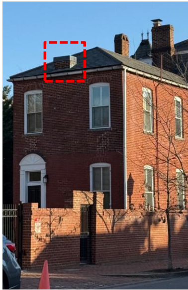
Photo 1: Existing chimney to be extended.
