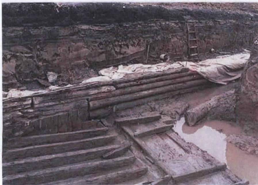
Figure 23: Bulkhead Repairs Overlying a Barge (Engineering Science 1993)
