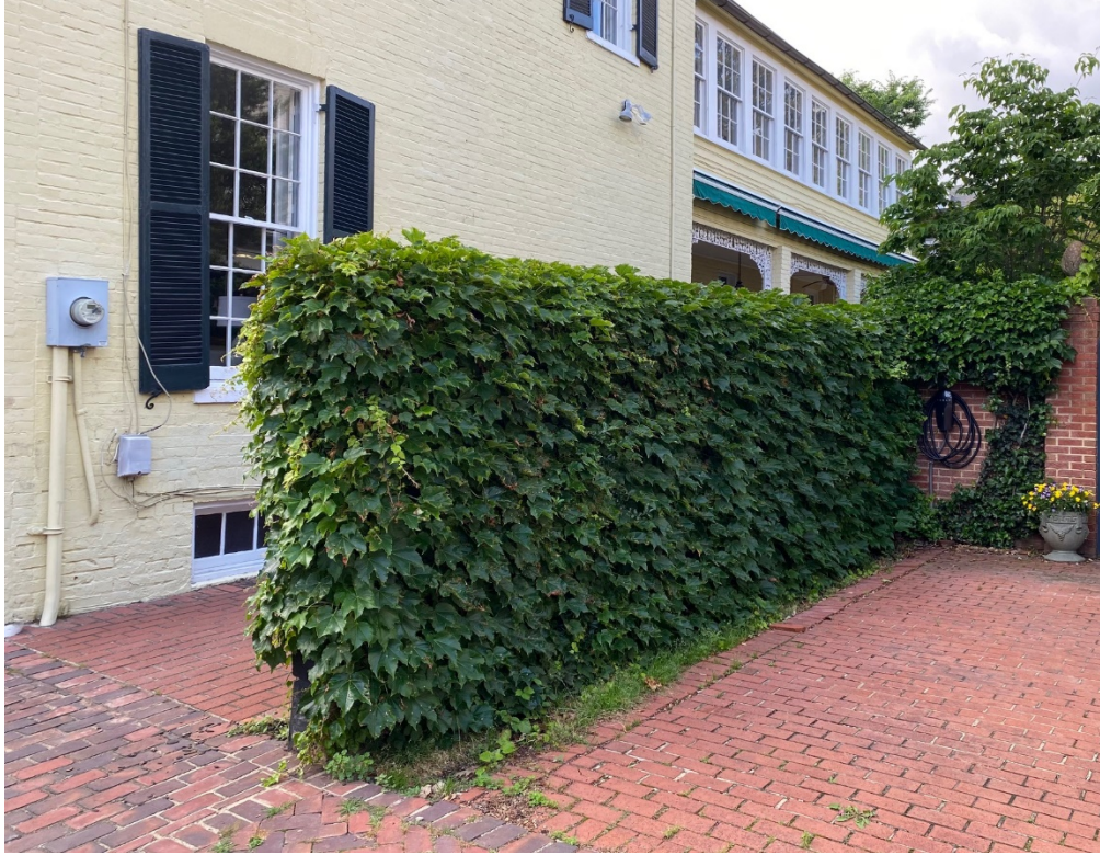
407 / 411 Prince Street Driveways: Masonry Dividing Wall with Ivy
