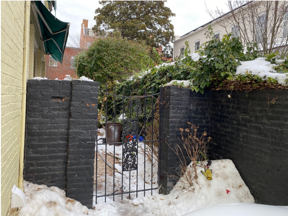
411 Prince Street: Masonry Wall & Iron Gate attached to Dividing Wall
