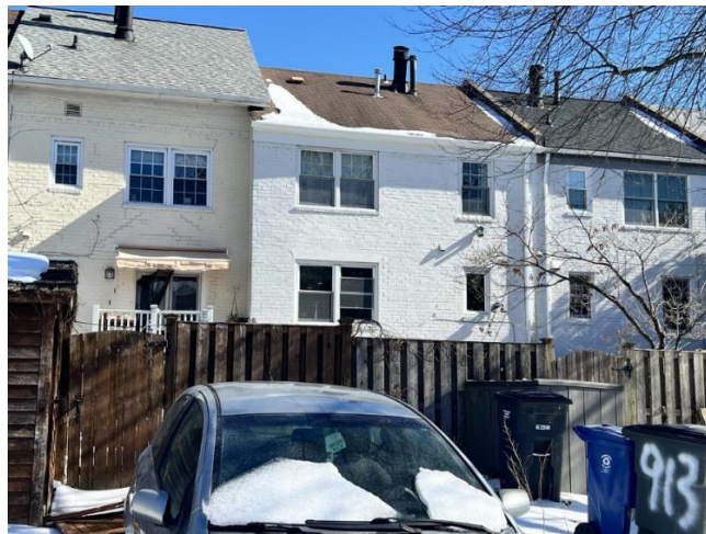
Figure 1. View of rear elevation from the public alley.
