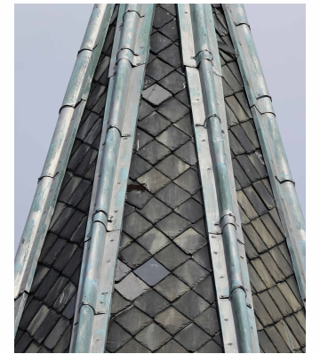
3 DIAMOND SHAPE SLATE ROOF TILE TYPE B
