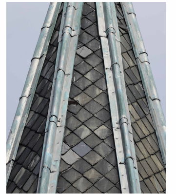
3 DIAMOND SHAPE SLATE ROOF TILE TYPE B
