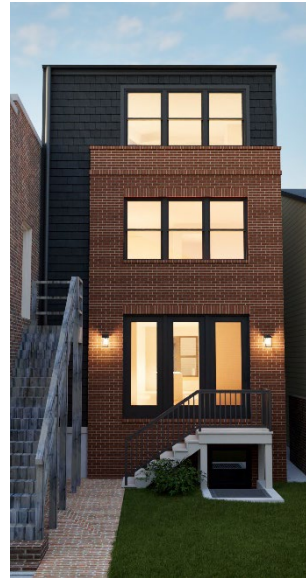
Figure 6: View of rear at sunset.
